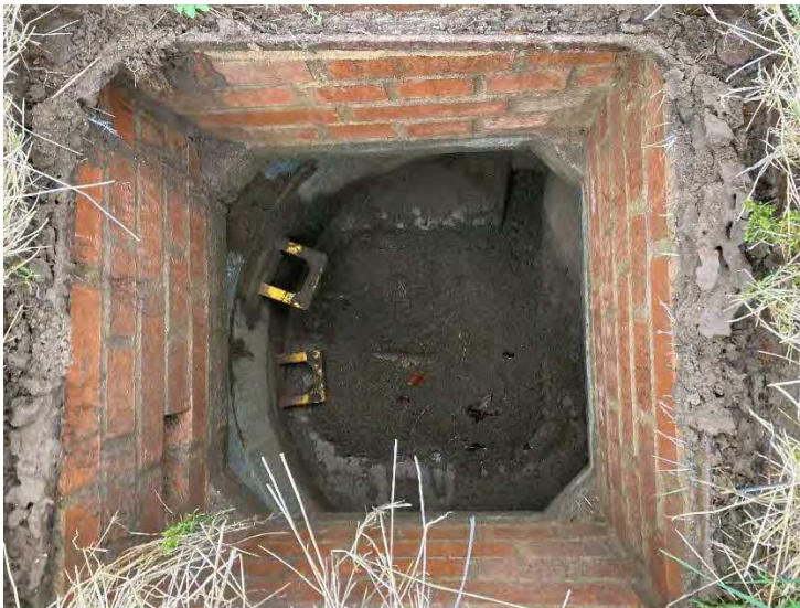
Figure 8-1: View of existing drainage
