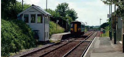
KENNETT RAILWAY STATION
