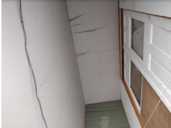
Figure 7. View of the internals showing no roof void.
