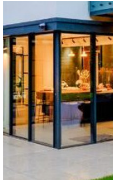
New glazed doors to extension in black aluminium.
