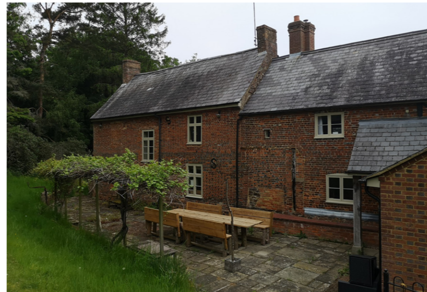
1 - View of Rear facade
