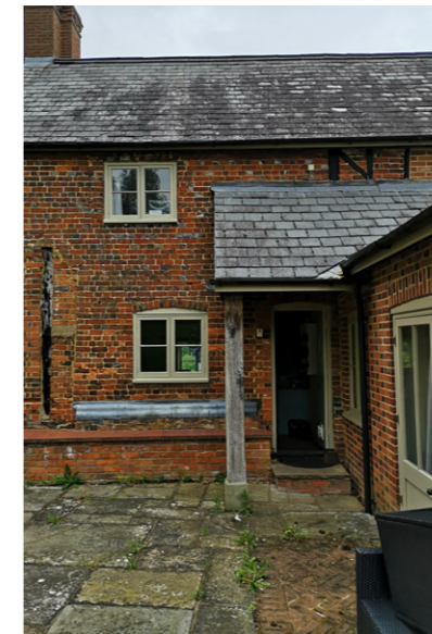
2 -Rear entrance canopy
