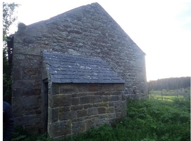
East gable of the Outbuilding 1 with small lean-to
