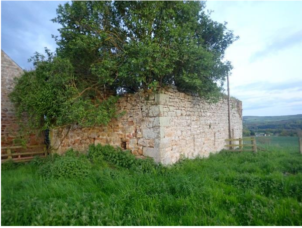
Outbuilding 2 from the northwest
