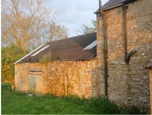
Outbuilding 1 from the northwest
