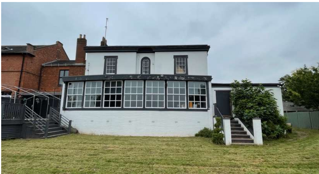
Figure 10 Existing rear (south) elevation of The Beeches.
