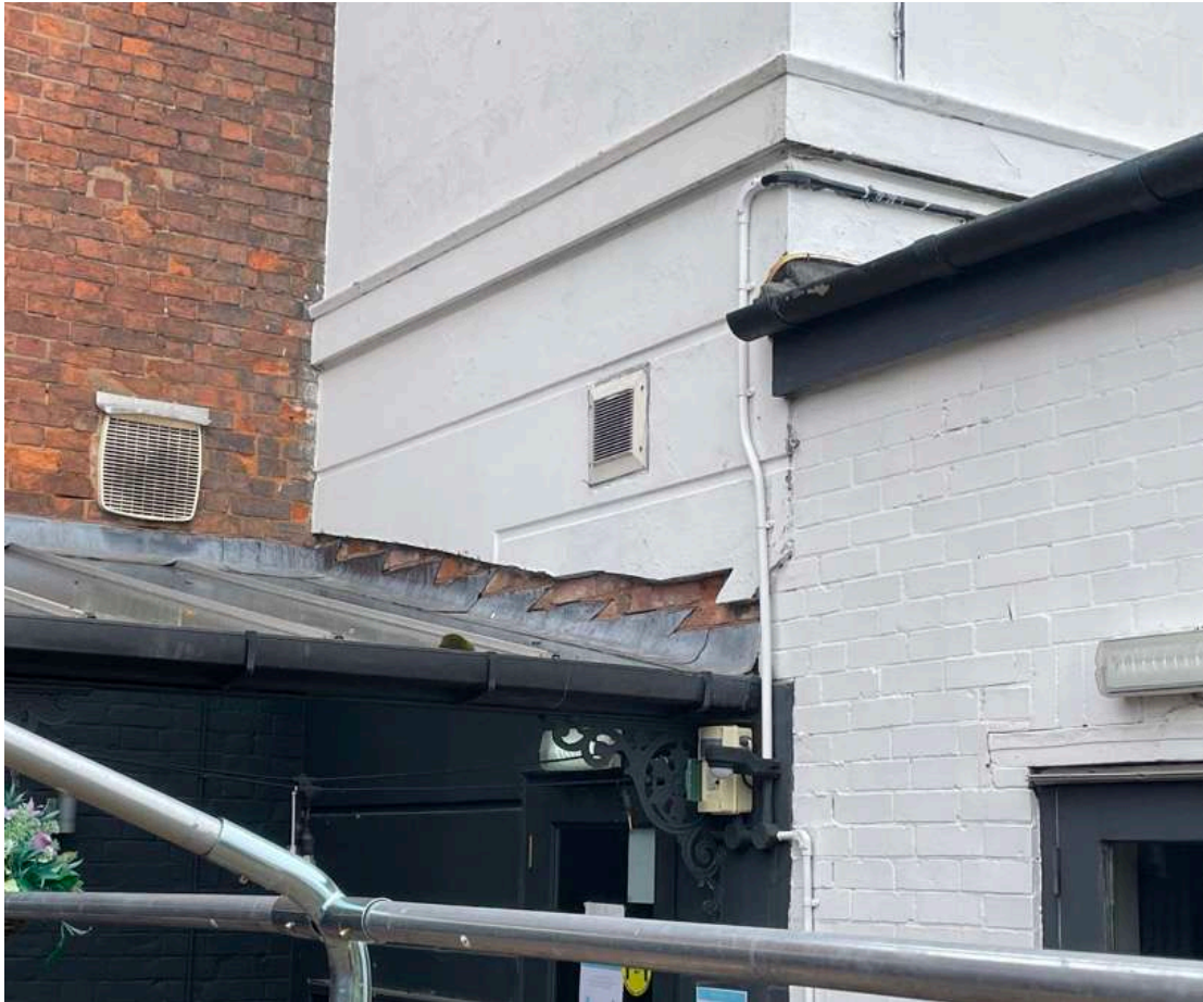
Figure 15 West elevation showing the brick 19th extension (left) to the original building (centre), the removal of original stucco facing for the addition of a glazed extension, and a modern painted brick extension (right).
