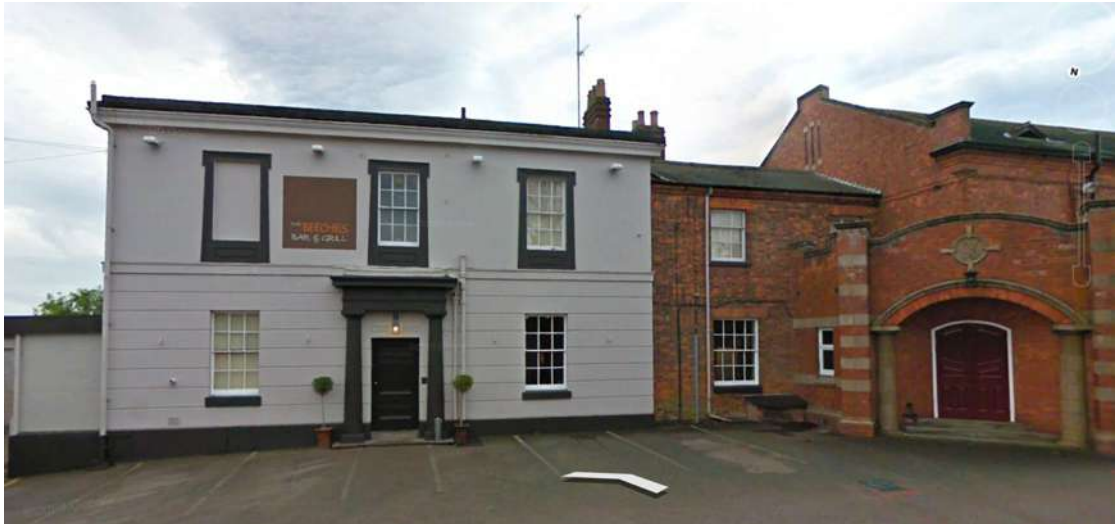
Figure 19 View south-west towards the Fentham Institute from the car park of The Beeches. Source: Google Earth.
