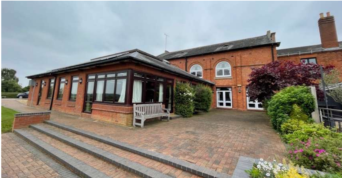
Figure 9 Modern single storey extension off the south elevation of the Fentham Institute community hall is not included in the local listing.
