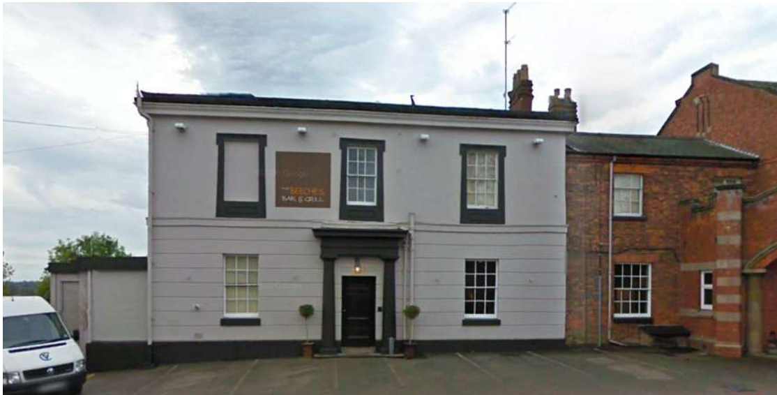
Figure 5 Grade II listed former Fentham Club with adjoining two storey brick extension to west (right) and later single storey kitchen extension to east (left). Source: Google Earth.
