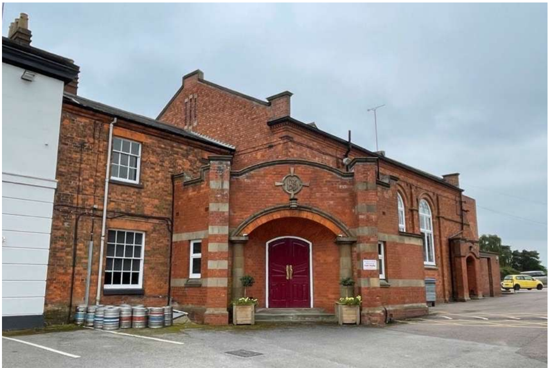
Figure 8 Locally listed Fentham Institute community hall adjoining The Beeches (grade II), viewed looking south-west.
