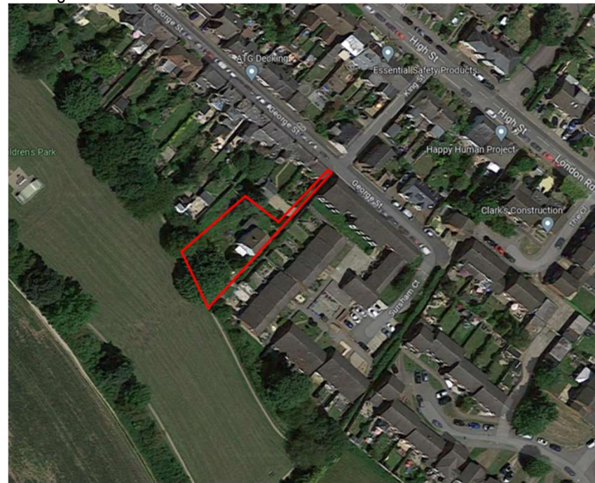
Site location (highlighted in red) – Aerial view (google maps)
