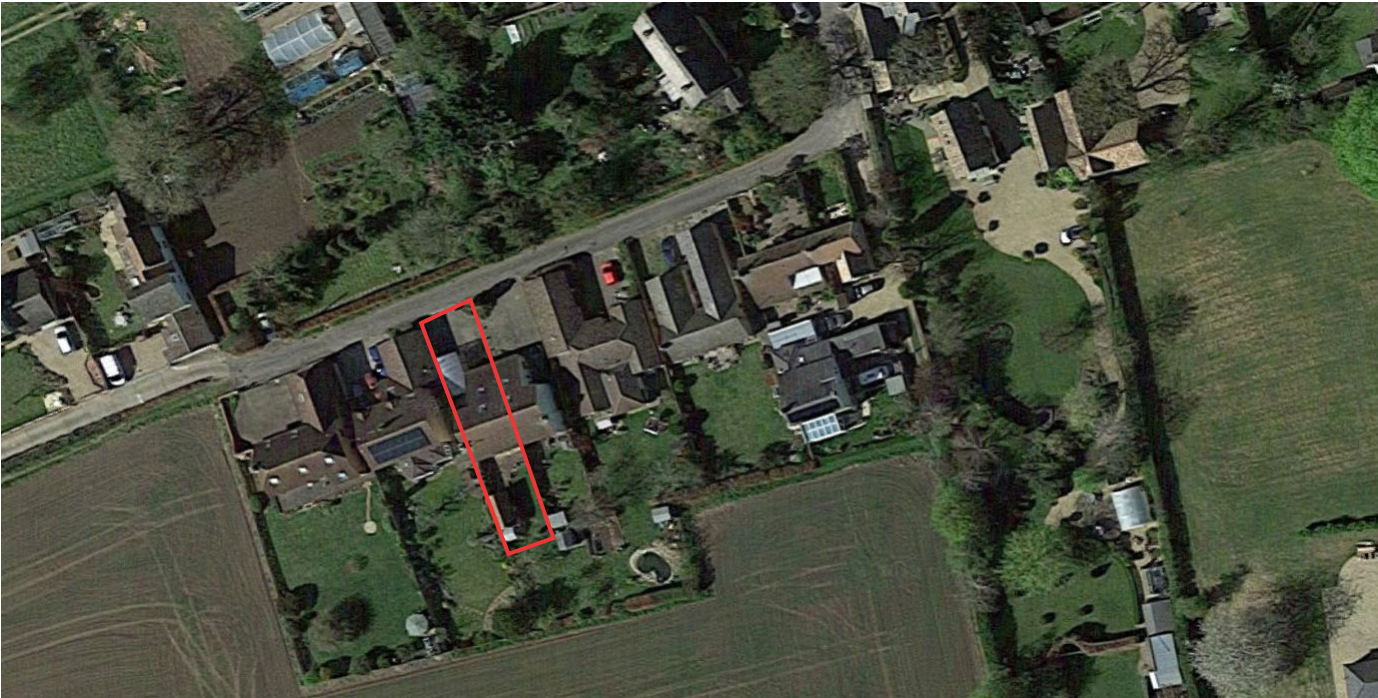
FIG 1: Aerial view of site
