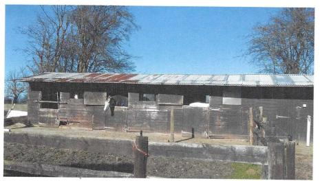
Old-fashioned and damaged Linear wooden stables block comprising 1 feedroom (RHS) and 3 stables. Currently these buildings are dangerous and horses can only stay in them during the day when someone is here in case of collapse. Some illustrations of damage shown below:
