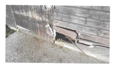
Left hand side stable damage to front and door not functioning
