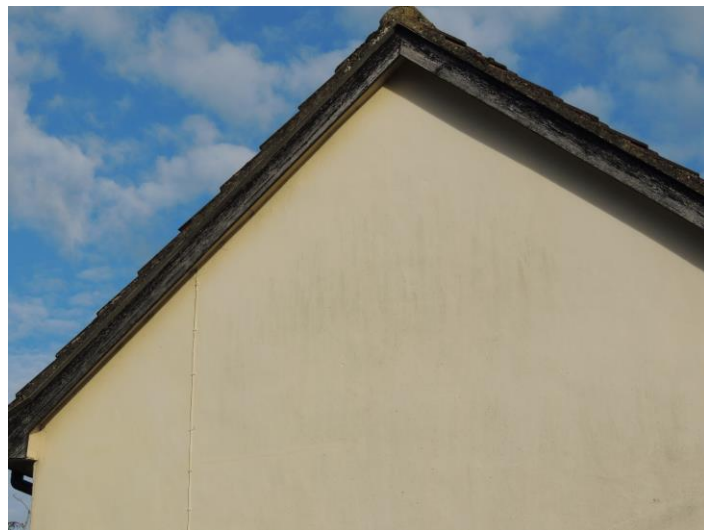
Photo 11: There was a tight seal to the gable of Granary Cottage
