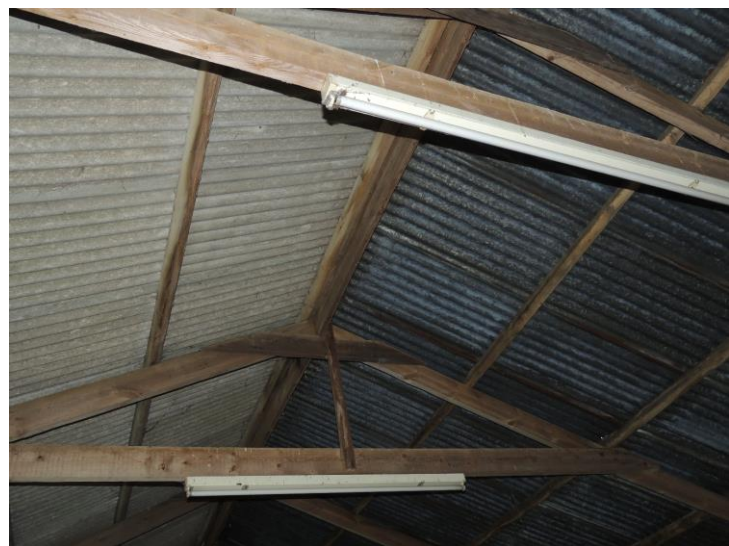
Photo 9: The roof had no features that might be occupied by bats
