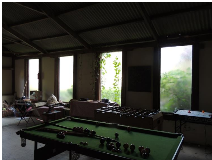
Photo 8: Showing windows in north wall
