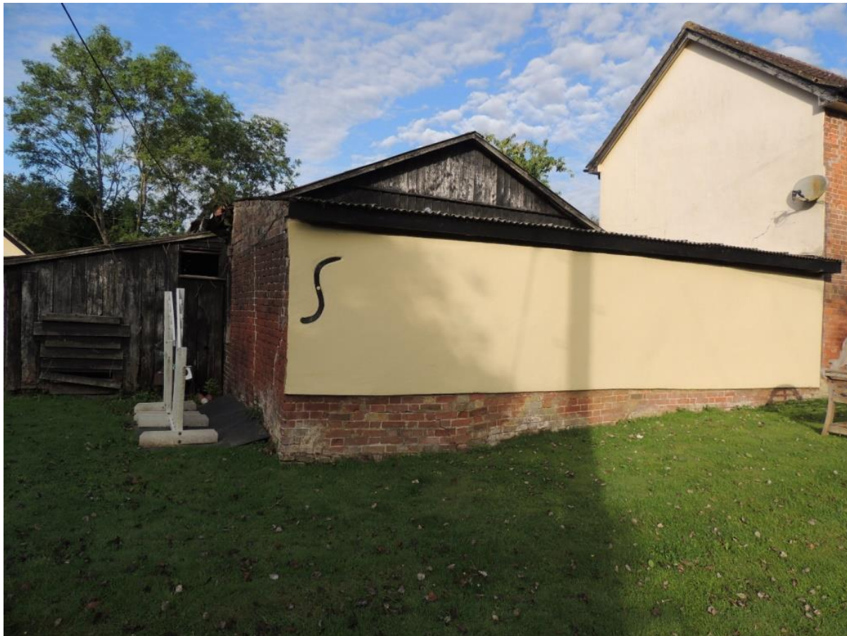
Photo 1: Eastern elevation. The southern gable wall of Granary Cottage is shown.
