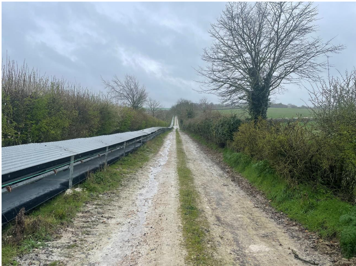
Photo 1 Conveyor and Maintenance Access Road
