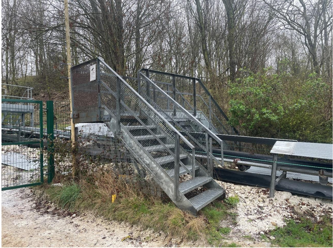
Photo 3 Footpath 43 Bridge Over Conveyor
