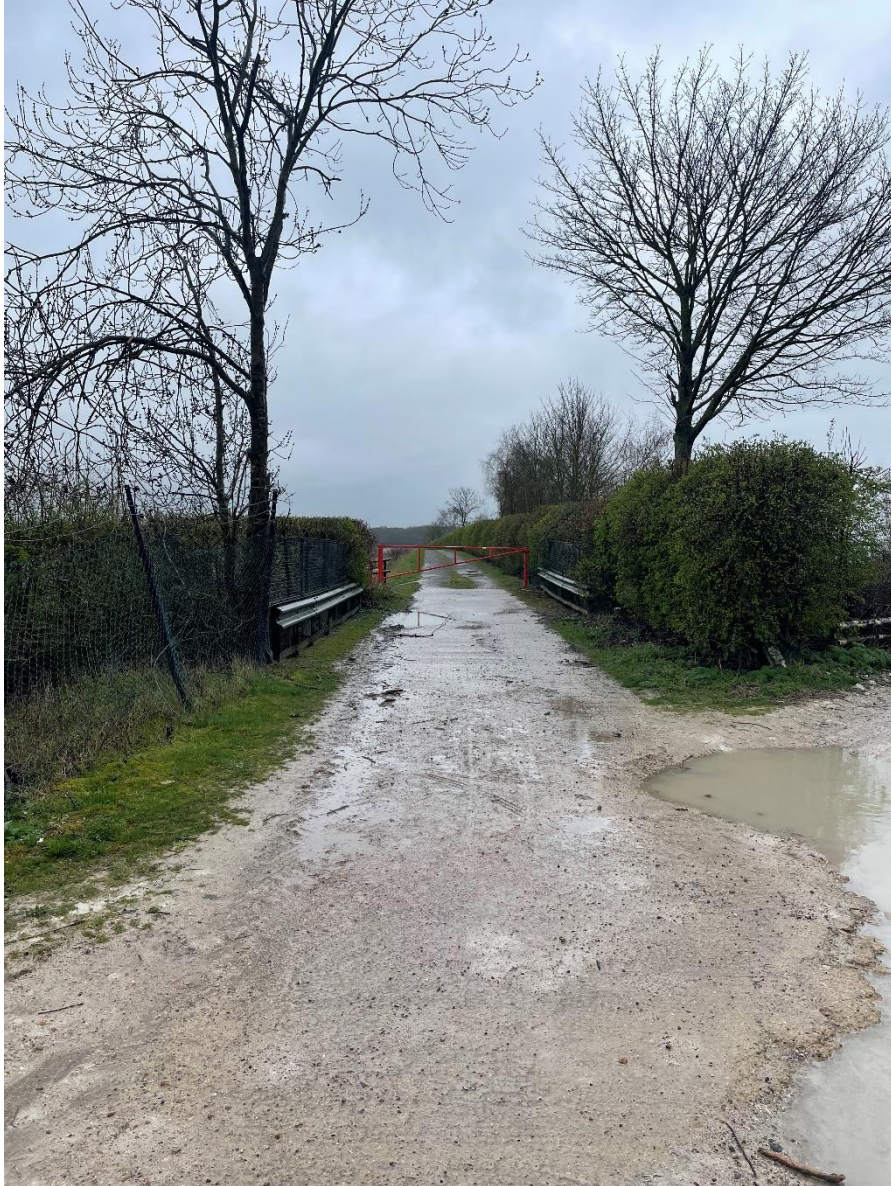
Photo 3 Point at Which Bridleway 46 Crosses the Access Road
