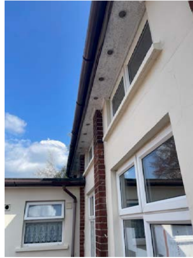
Main School Building - sealed soffits
