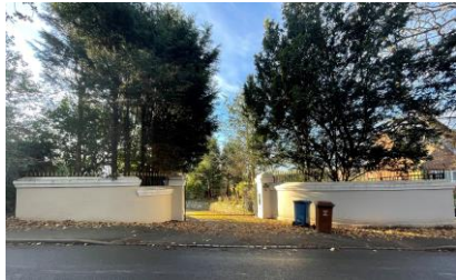
05 View 1 - Main site entrance/egress.
