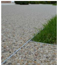
46 Permeable resin bound drive
