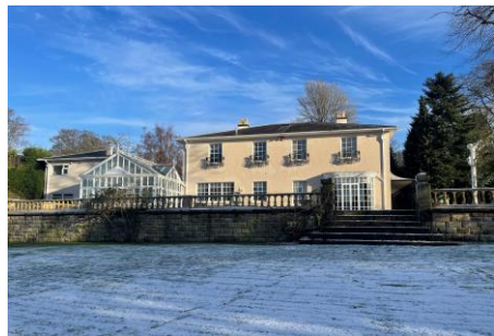
09 View 5 – Rear of dwelling with raised terrace in foreground.
