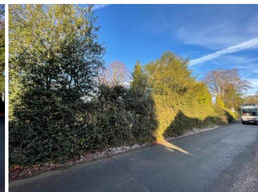
14 View of boundary at south-west corner.
