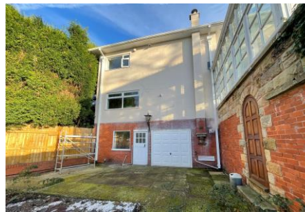
10 View 6 – showing rear of annexe and rear side of conservatory.
