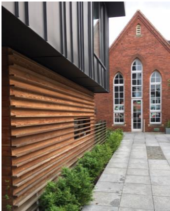
29 Combination of timber and standing seam cladding.
