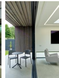
33 & 34 Proposed deep canopies with flat panel cladding (Equitone) & timber soffits.
