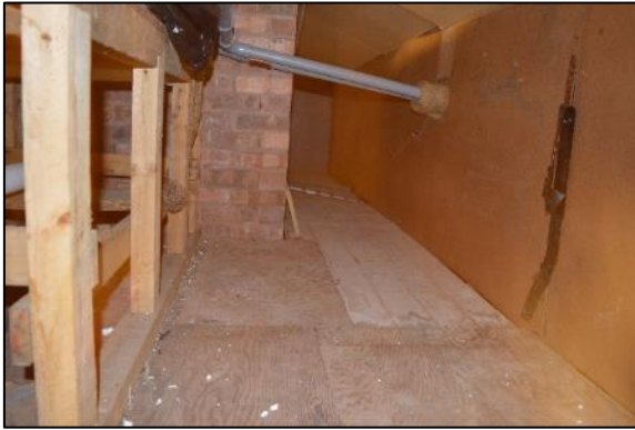
Figure 18: Internal crawl space of B1a
