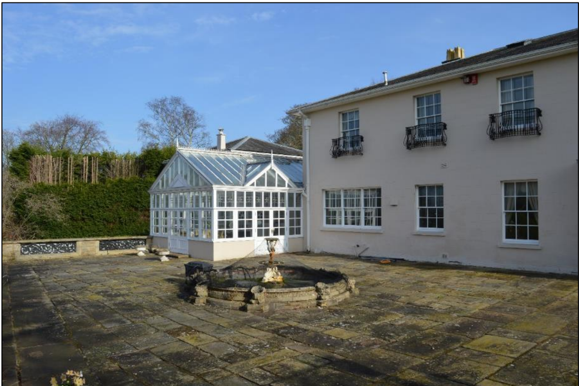
Figure 15: Western elevation of B1a and B1b
