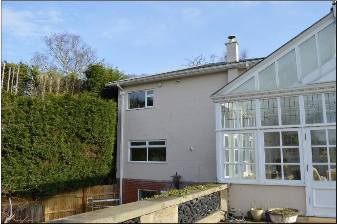
Figure 16: Western elevation of B1c
