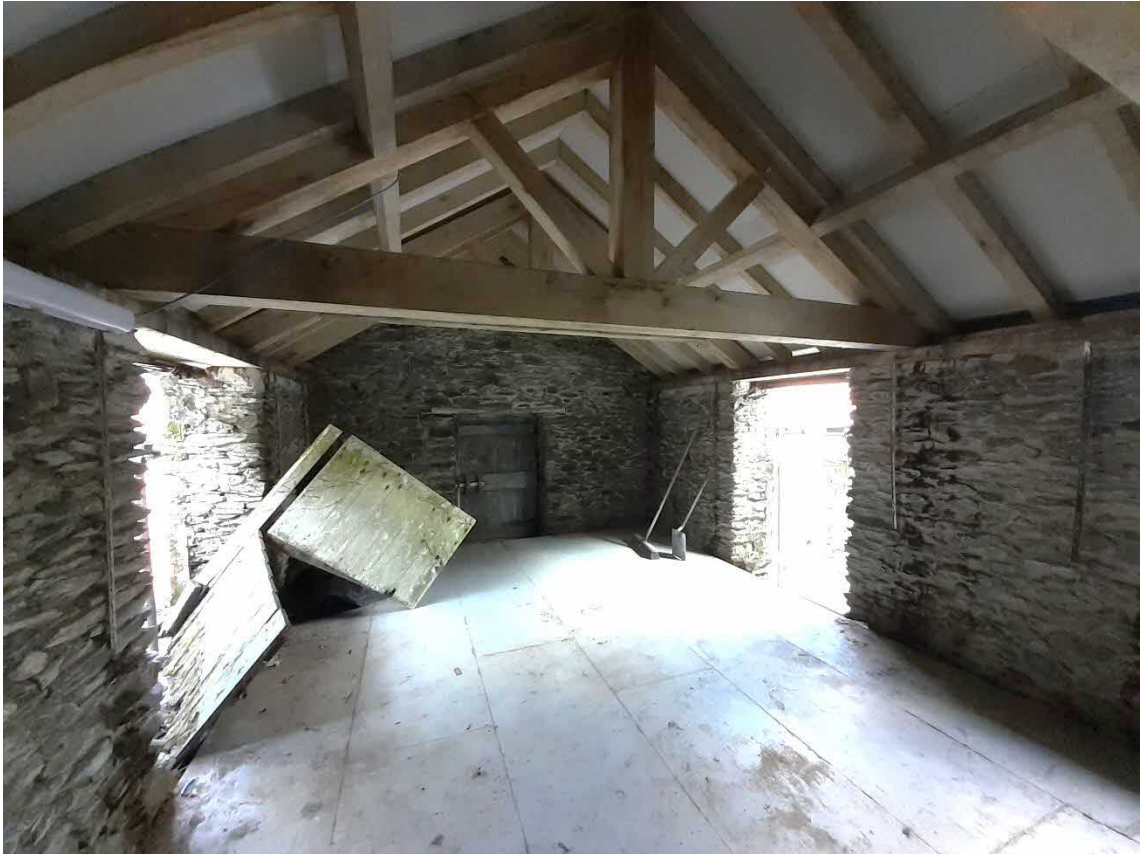
New traditional timber truss and purlin roof
