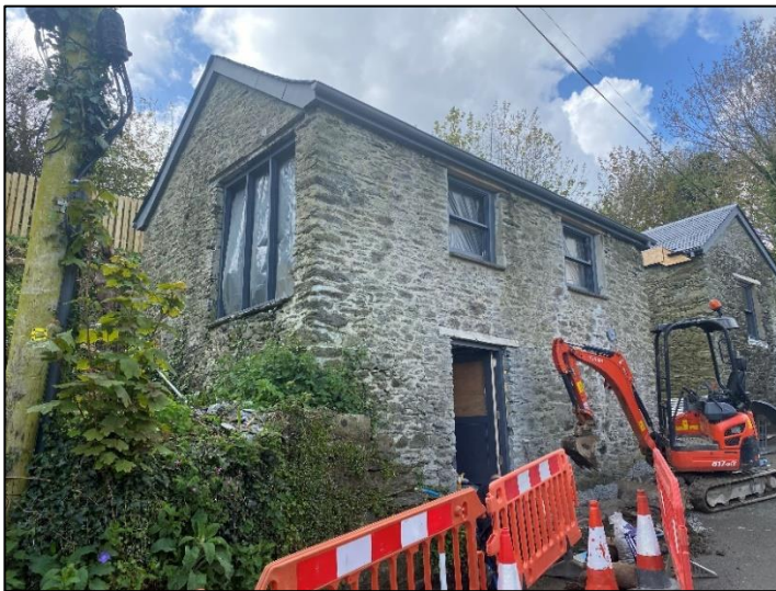
Photograph 1: Building 1 northern and eastern elevations
