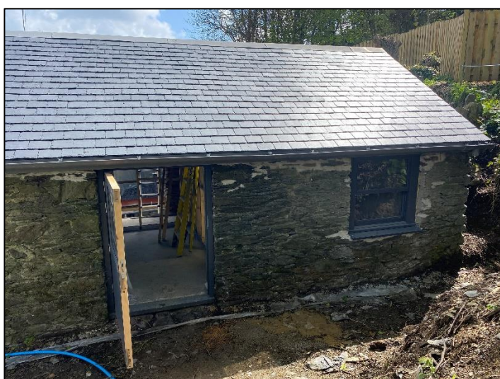
Photograph 4 – Building 2 western elevation
