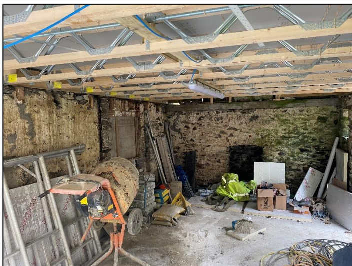
Photograph 5: Internal of Building 1 on ground floor
