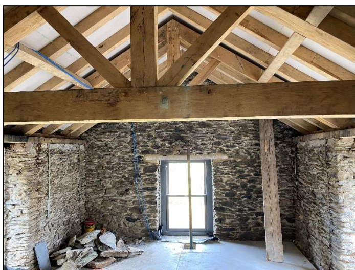
Photograph 6: Internal of Building 2 on first floor
