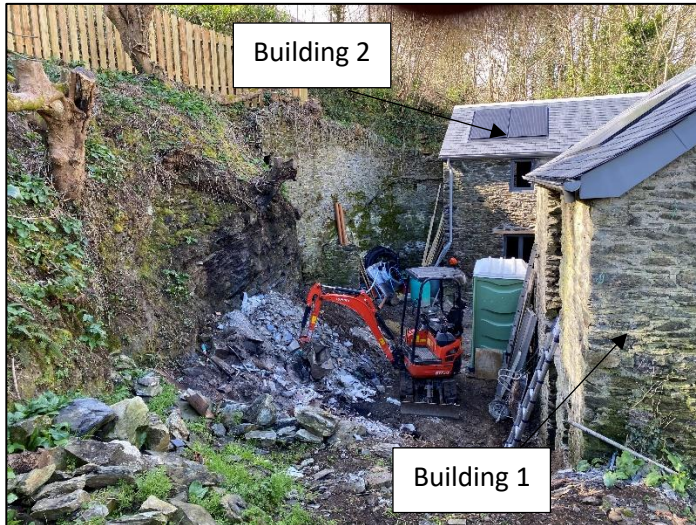
Photograph 7 – Outside space to the south of the buildings
