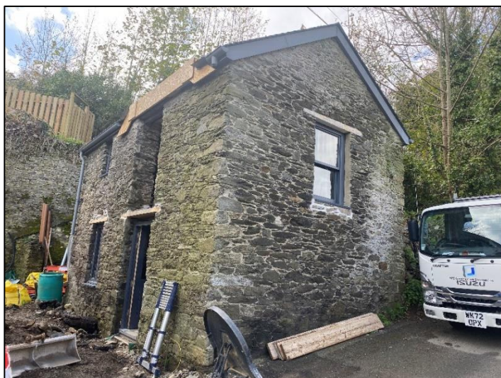
Photograph 2 – Building 2 northern and eastern elevations
