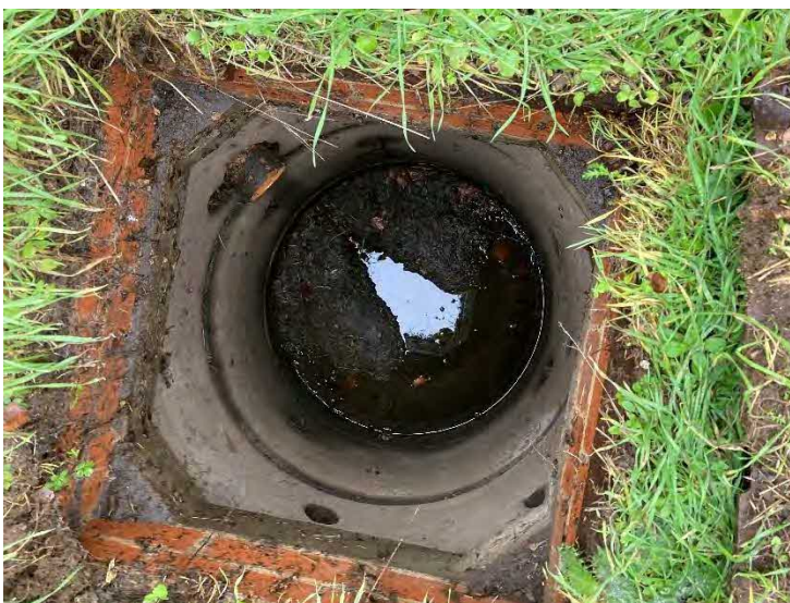
Figure 8-2: View of existing drainage
