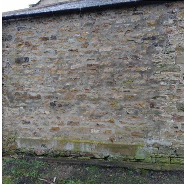
Figure 20. Cement mortar pointing to west wing west wall.
