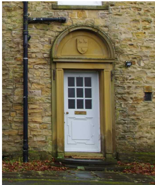
Figure 8. north elevation entrance door with Arms.
