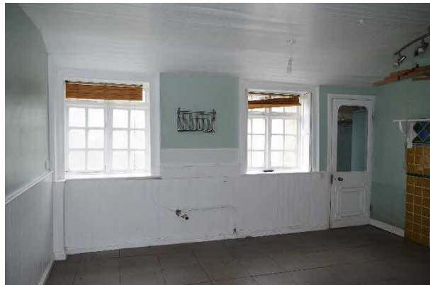
Figure 23. Existing kitchen timber boarded ceiling
