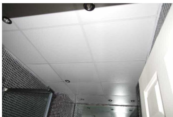
Figure 26. Modern suspended ceiling in Ensuite.
