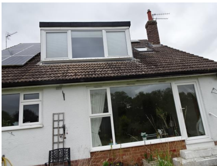
Rear elevation facing onto the river
