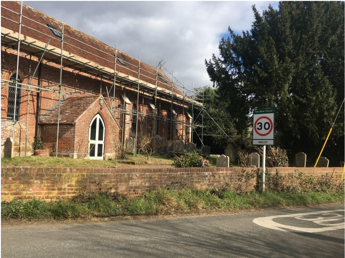
Figure 6: Exterior south elevation, south porch, and graveyard setting
