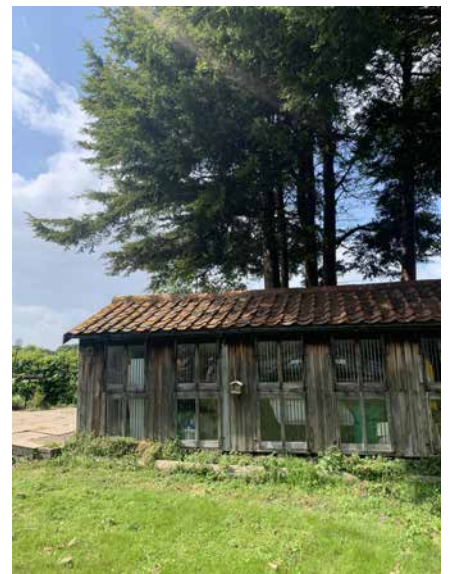
EXISTING OUTBUILDING & MATURE TREES TO N-E BOUNDARY
