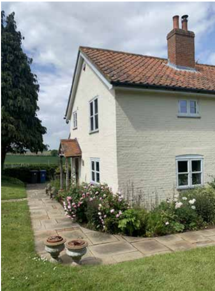
EXISTING DWELLING S-W CORNER
