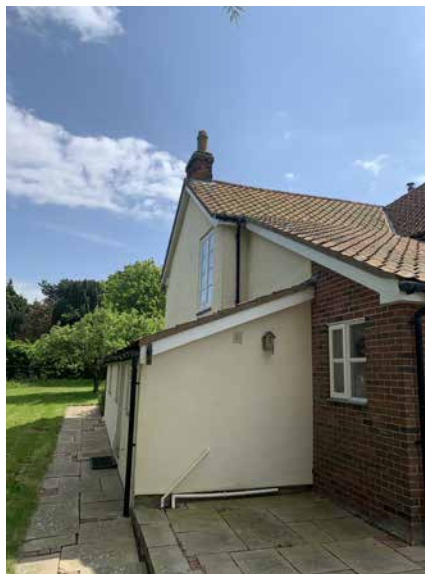
EXISTING EXTENSION N-E CORNER
