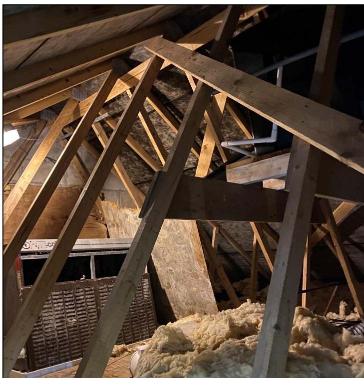
Photograph 4 – loft space of single storey building (TN3)
