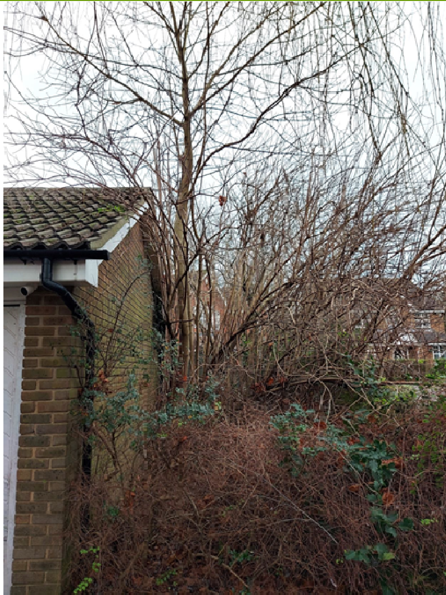
P5. The location of the group of trees (G1), growing immediately adjacent to the garage wall, is not sustainable and the group is recommended for removal for arboricultural reasons.
