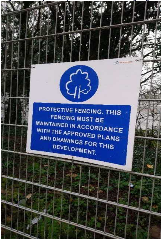
Fig 3 example of protective fencing sign.
