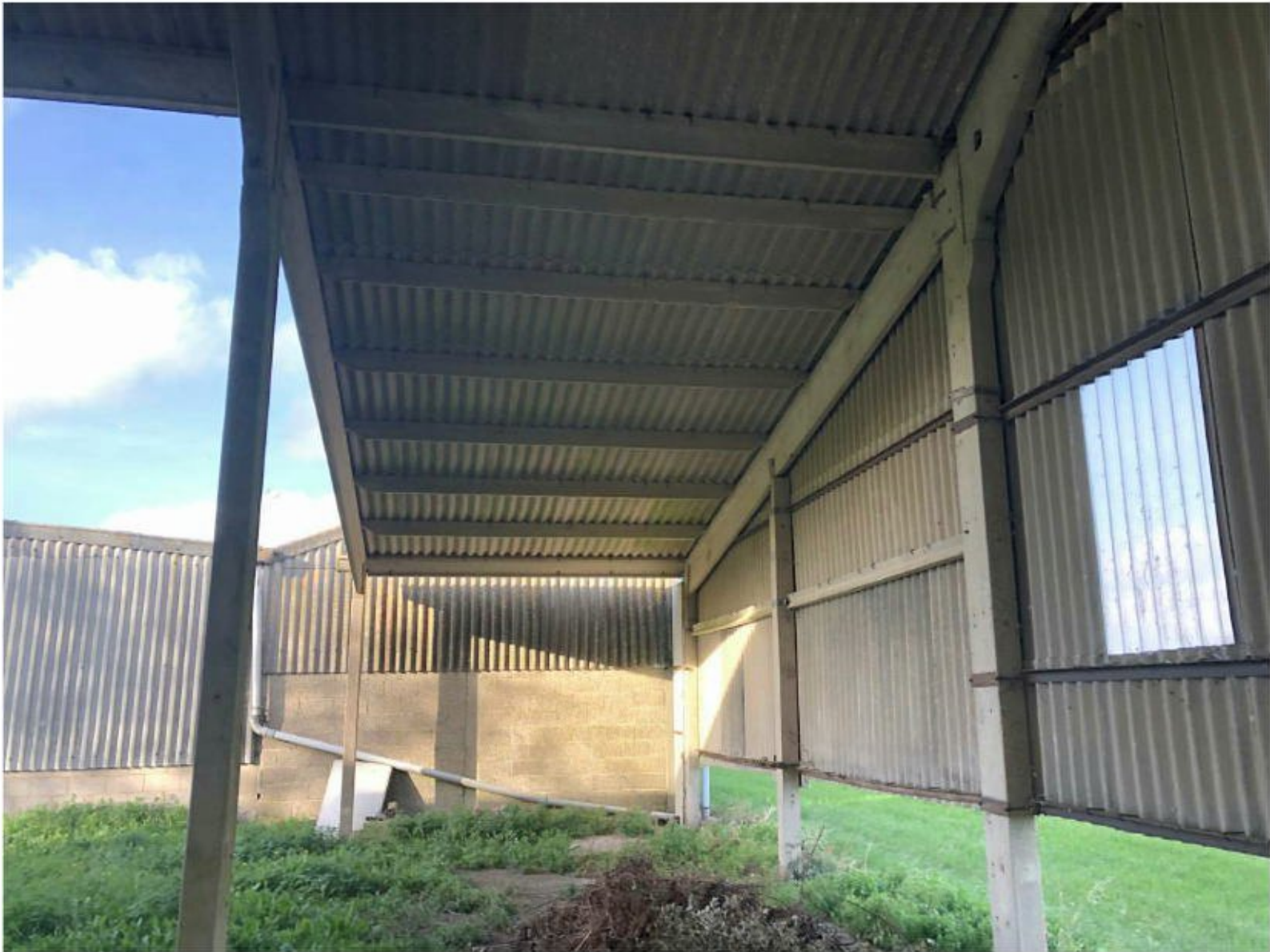
View on lean-to to north side of barn showing structure
