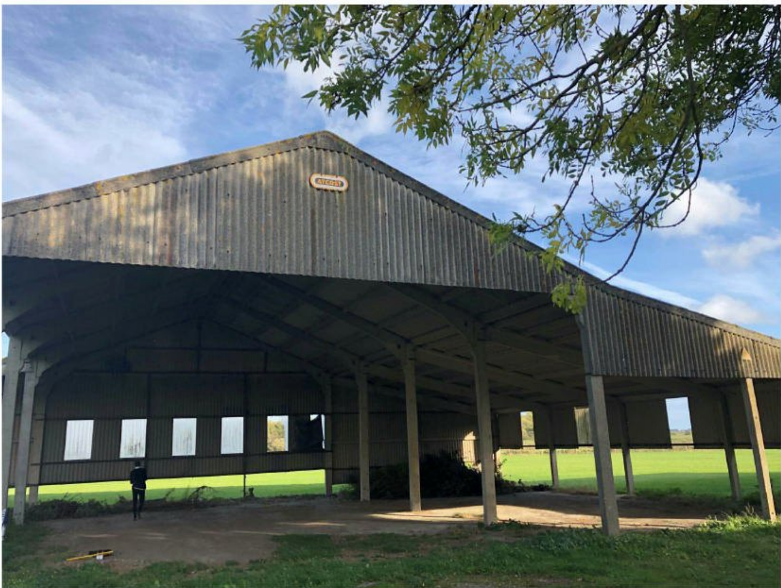
View on bean showing concrete frame structure
