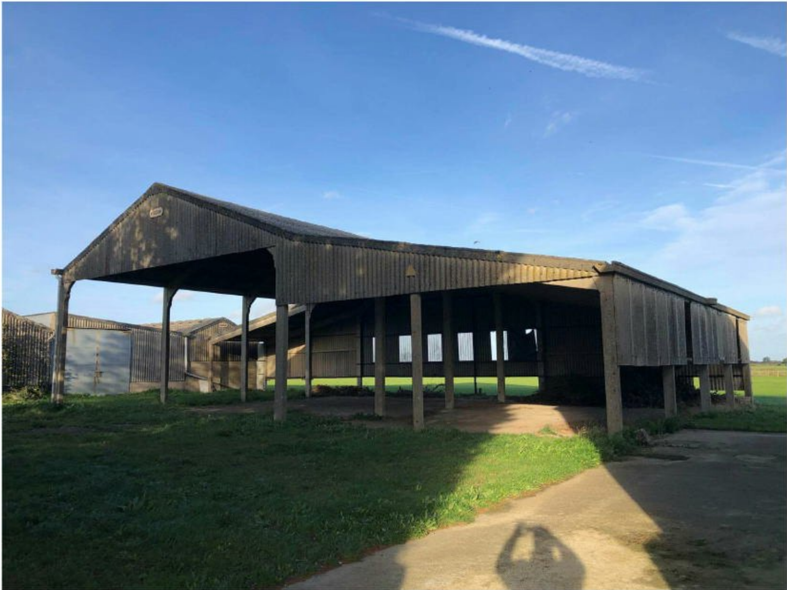
View on front of barn from south west
