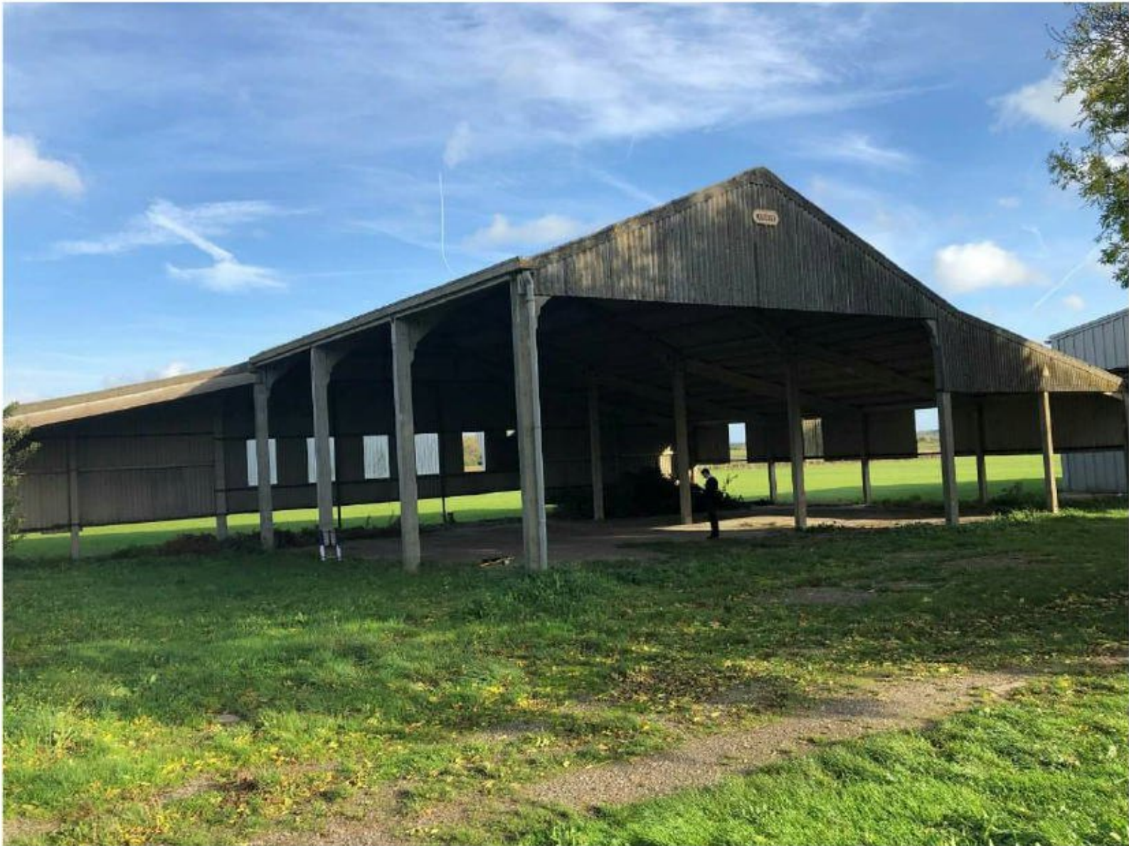
View on front of barn from north west
