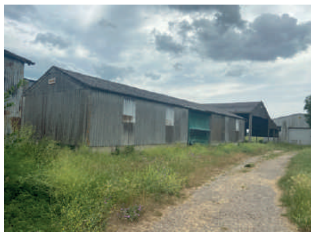
Fig 6 Existing barn adjacent to the proposed barn.
