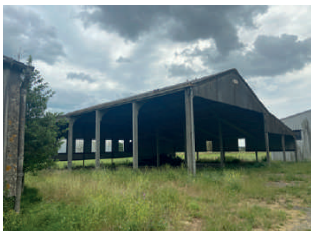
Fig 7 Existing photograph of the Atcost barn to be converted.
