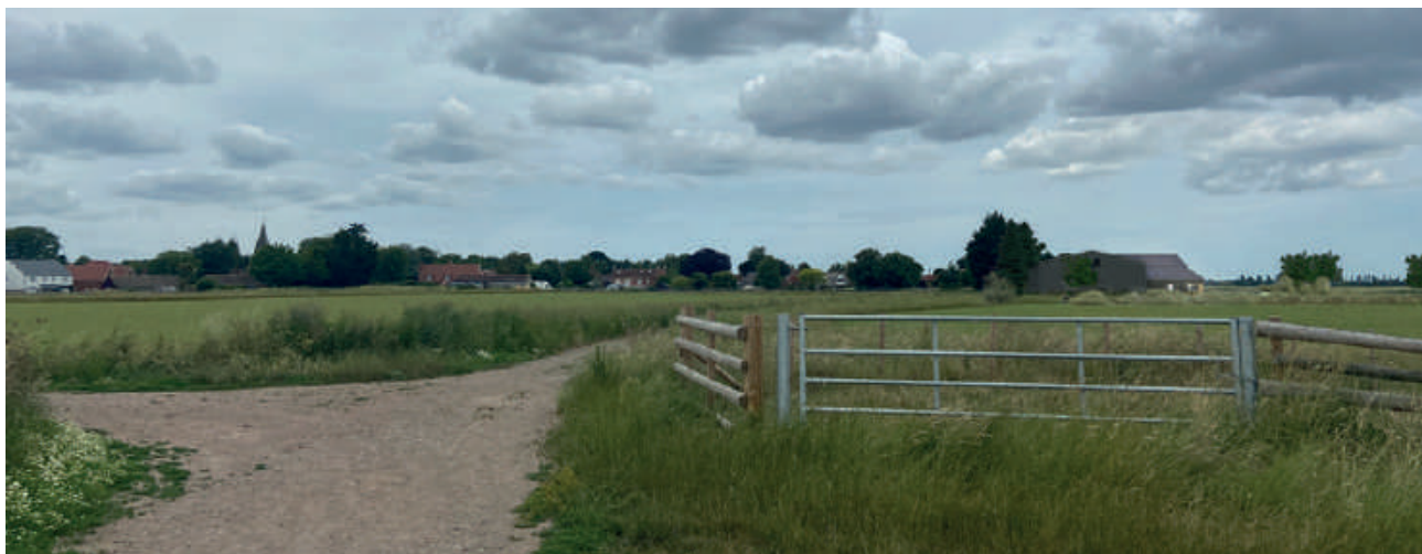
Fig 20: View from the south east corner of the site with the proposals in context with Worth.
