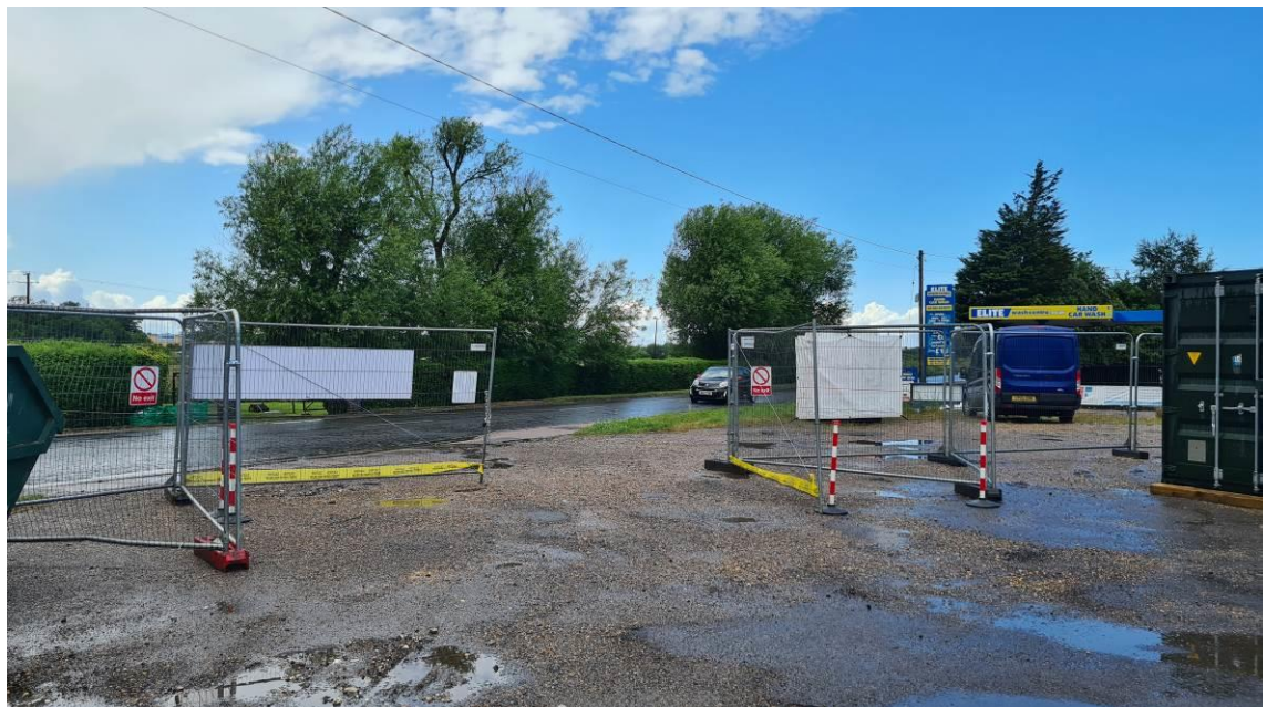
Figure 4: Site Access Point Viewed from within The Site.
