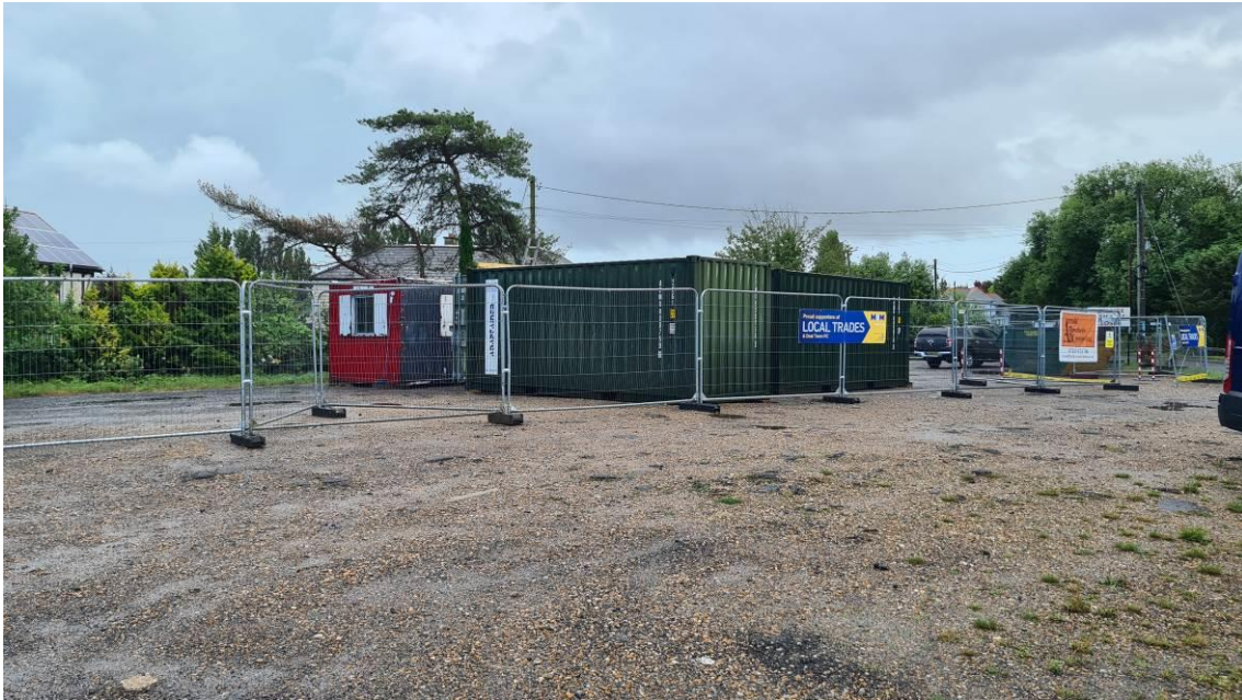
Figure 8: Materials Storage / Construction Compound Looking Southeast.
