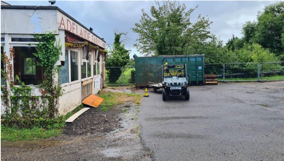
Figure 9: Deployment of Skips on Hardstanding for Soft Strip Arisings.
