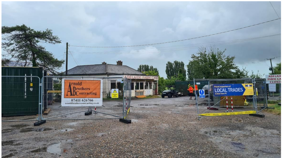
Figure 3: Site Entrance with Temporary Holding Area Off the Public Highway.
