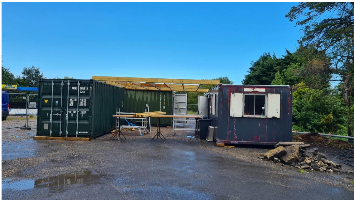
Figure 7: Compound Establishment in Progress with Materials Storage Facility.
