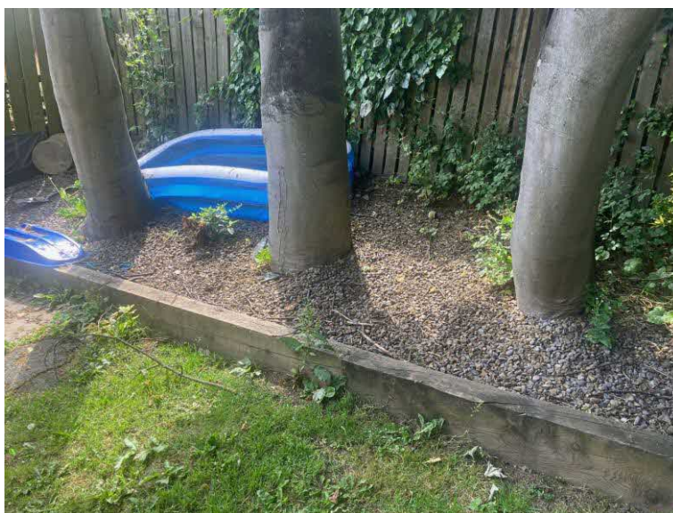
Photographs 2 – The base of trees T1 to T3 (growing in a raised bed)
