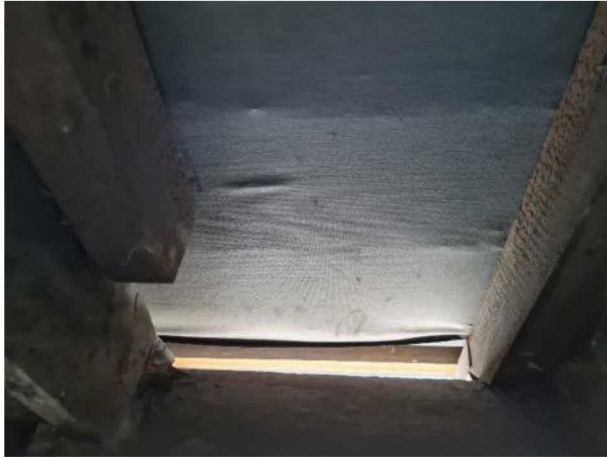
Figure 30: B3 - internal - light entering under eaves on south elevation
