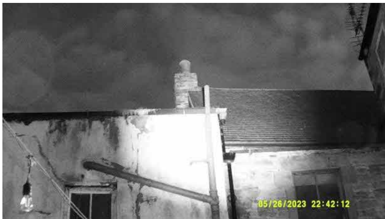
Figure 4: FOV IR camera - south elevation.
