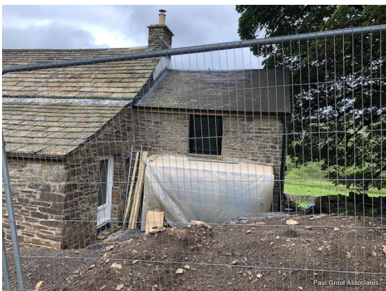
The west elevation (part)
