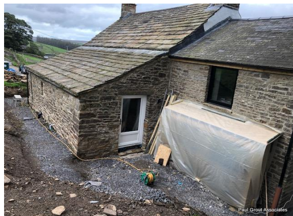
The west elevation looking south
