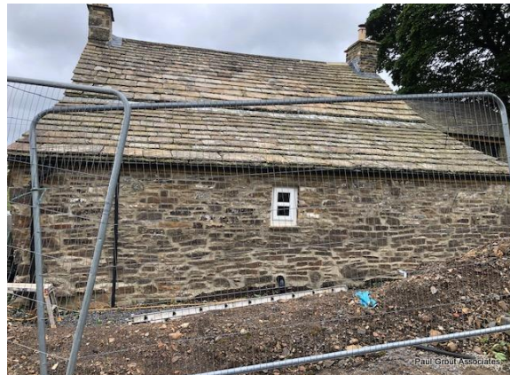
The west elevation (part)
