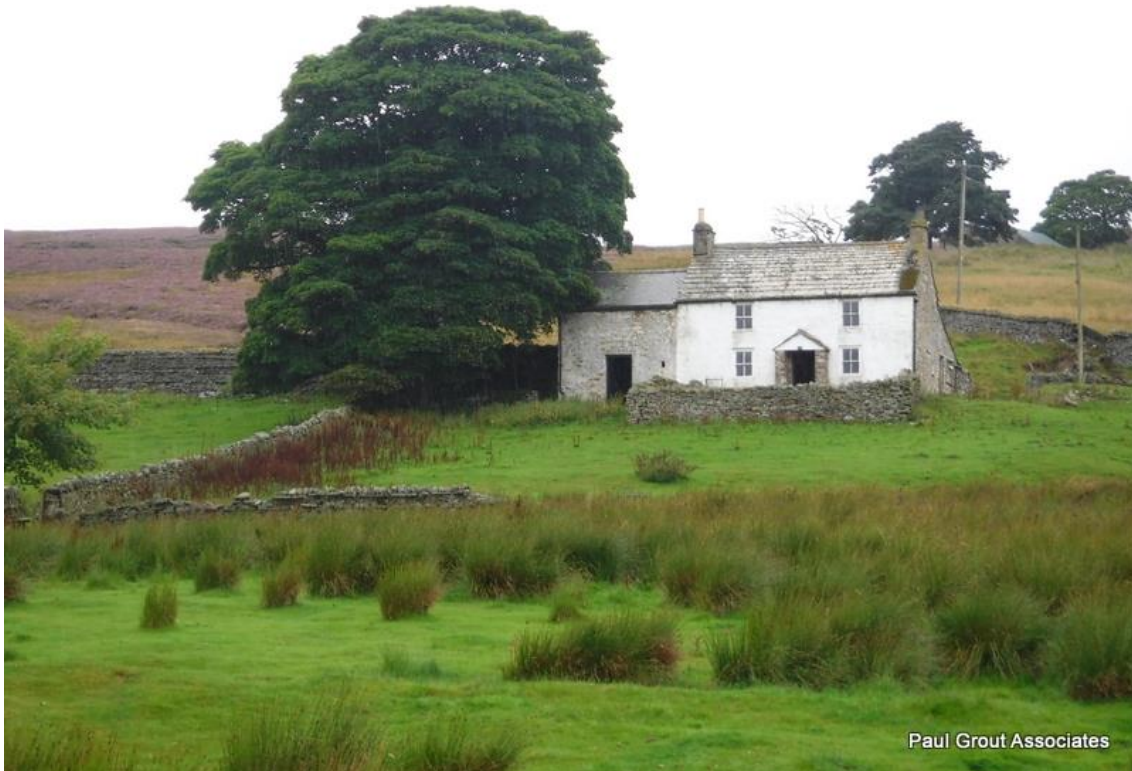
The existing house before the alterations
