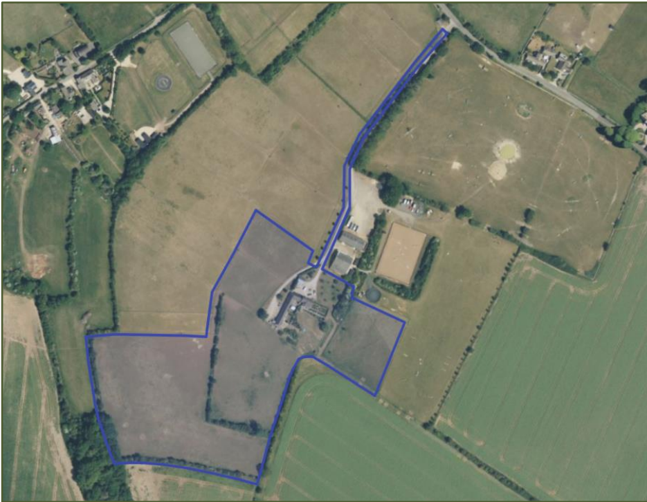
Figure 1 – Aerial image showing extent of New Barn Farm
