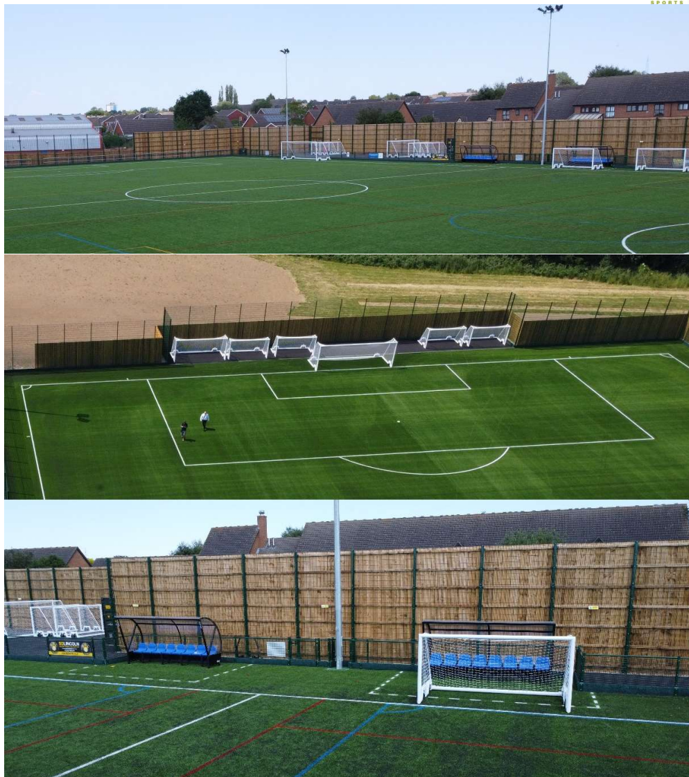
Examples of perimeter acoustic fencing
