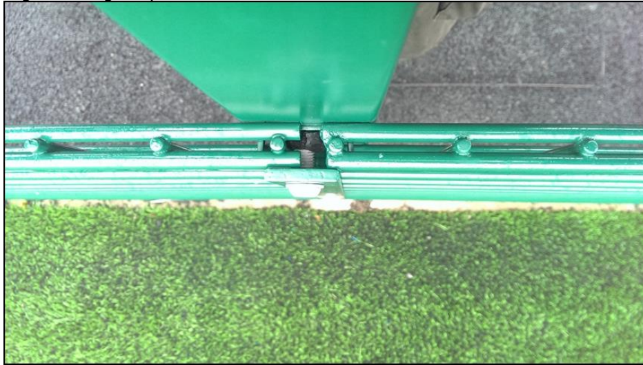
Figure 9: Image showing neoprene isolators
