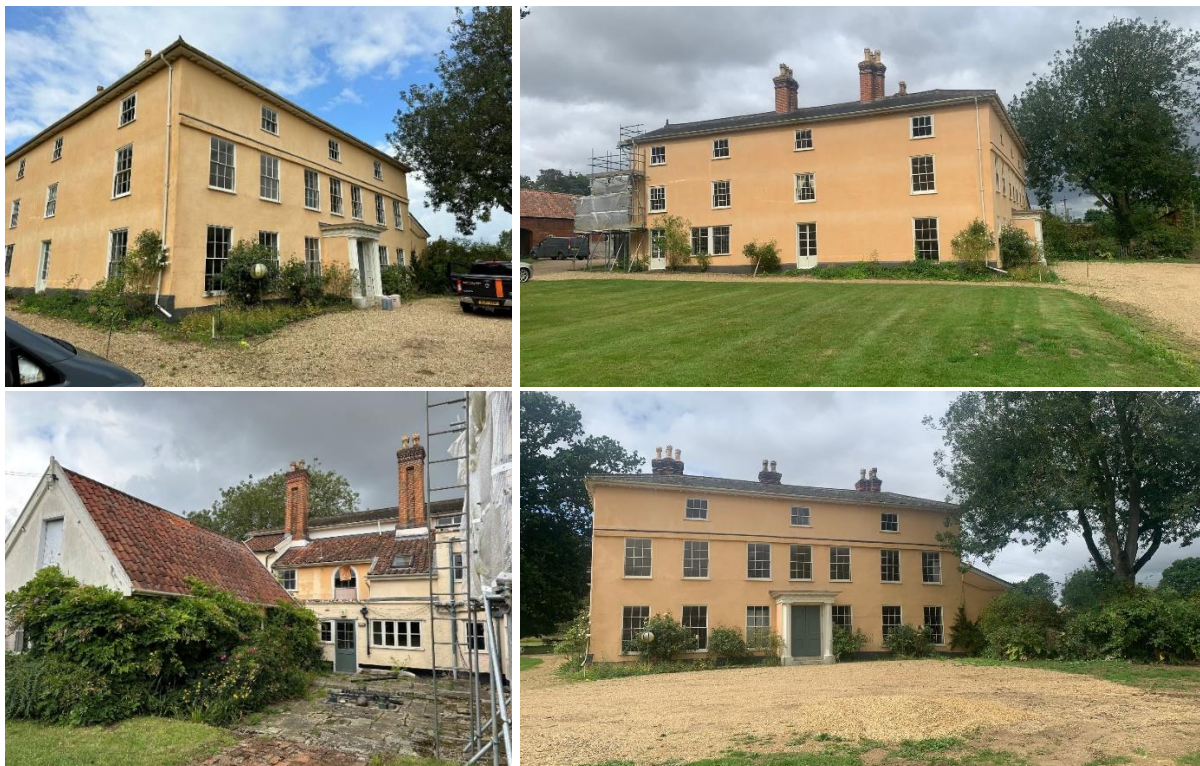
07-10 Views of the exterior of Buxhall Vale
