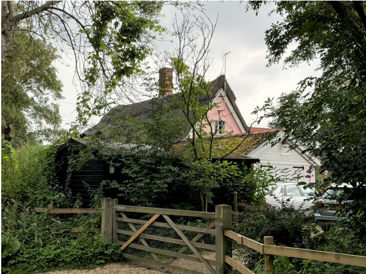
Rear of Lodge Cottage looking to east
