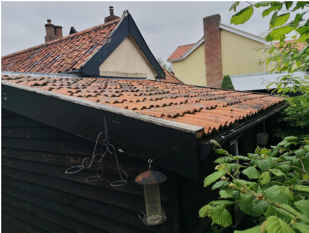
Photograph 4: Southern gable of outbuilding and pantile roof of store
