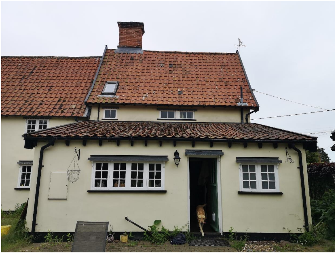
Photograph 1: Looking at single elevation extension to be extended
