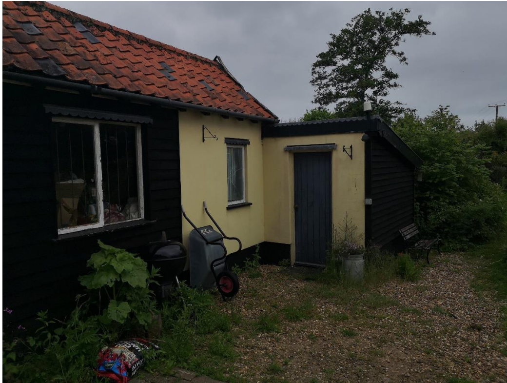
Photograph 3: Eastern side of outbuilding and gravel area for footprint of new extension
