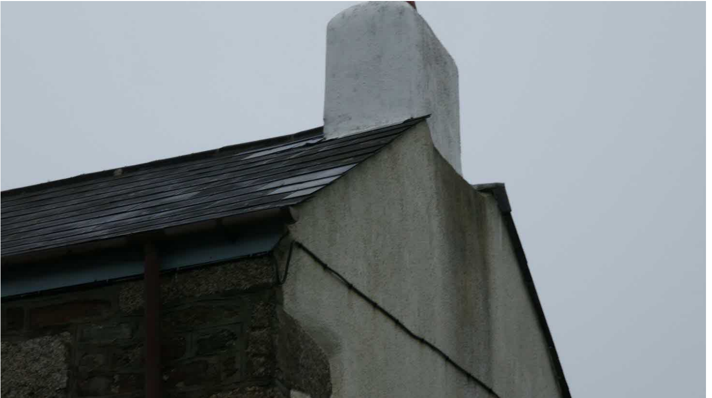
Figure 2. Eastern gable of the building.
