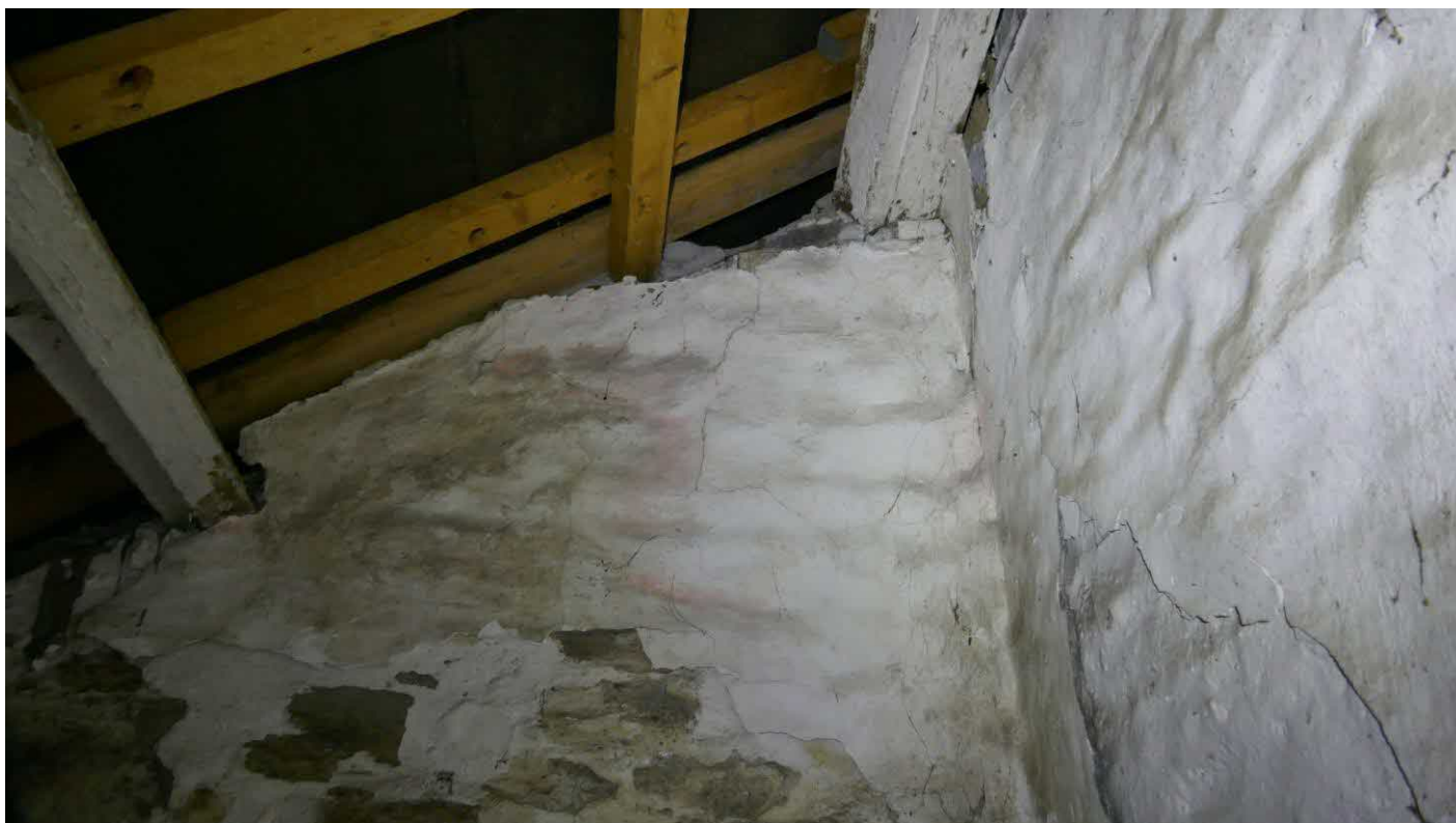
Figure 8. Roof void above the utility room on the north side of the building.
