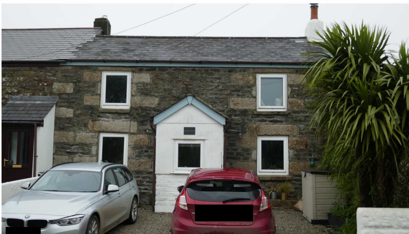
Figure 1. Southern aspect of the building.
