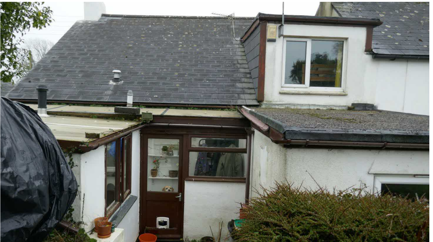
Figure 3. Northern aspect of the building.
