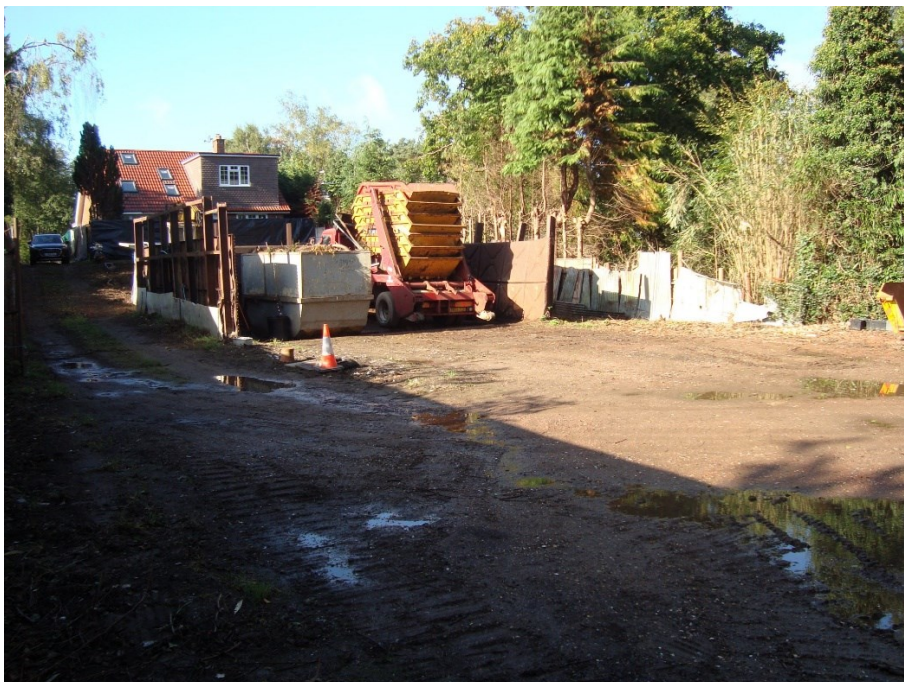
Image 03: View towards the top of the site
