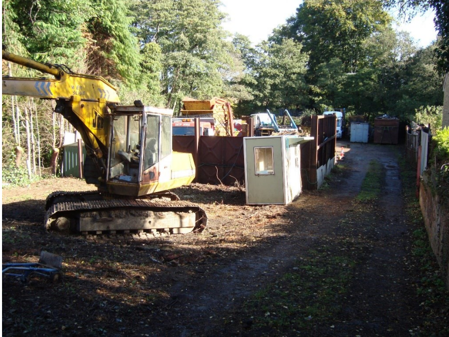
Image 02: View towards the rear of the site from the driveway
