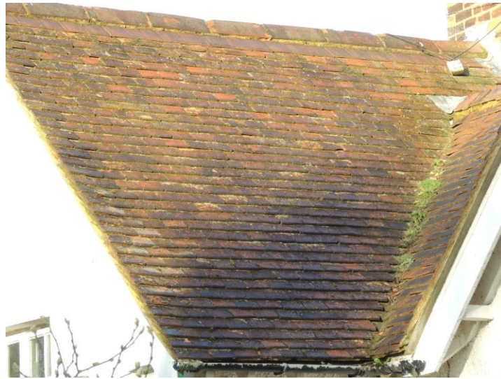
Photo 10: Note tight seal to roof tiles
