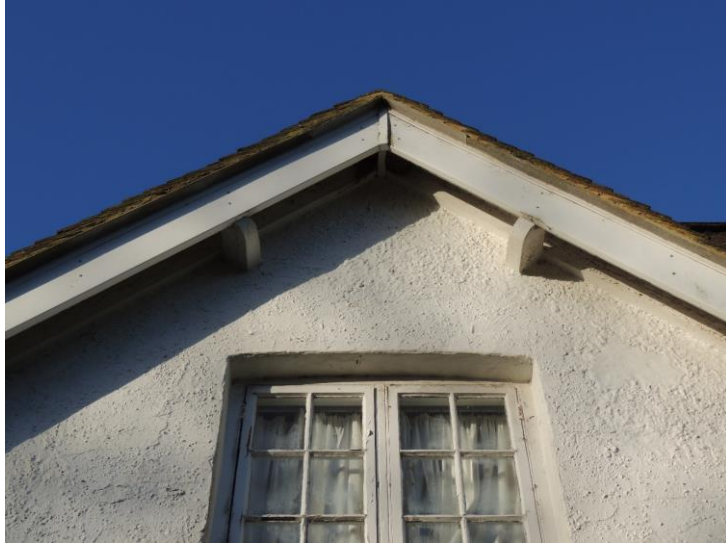
Photo 7: Note tight seal to gable
