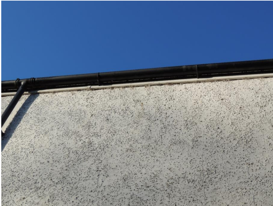
Photo 13: Note tight seal to fascia board of flat-roofed section of building
