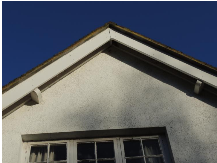
Photo 8: Note tight seal to gable
