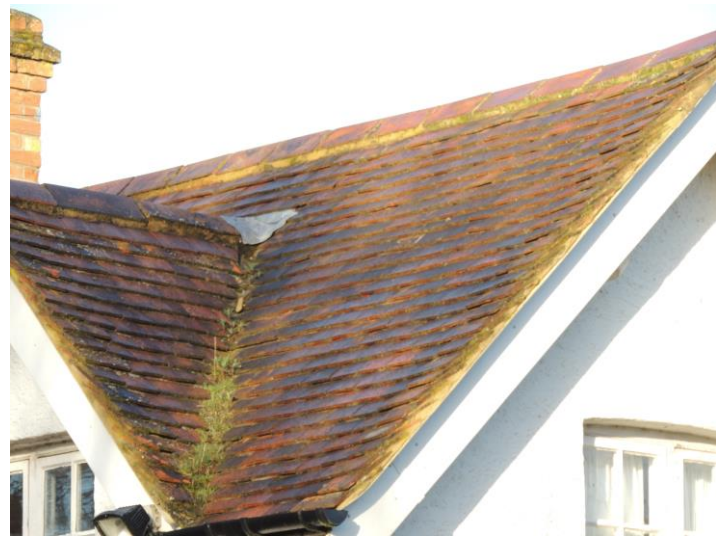
Photo 11: Note tight seal to roof tiles
