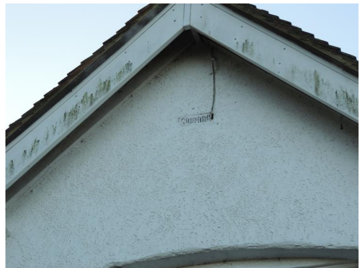
Photo 9: Note tight seal to gable
