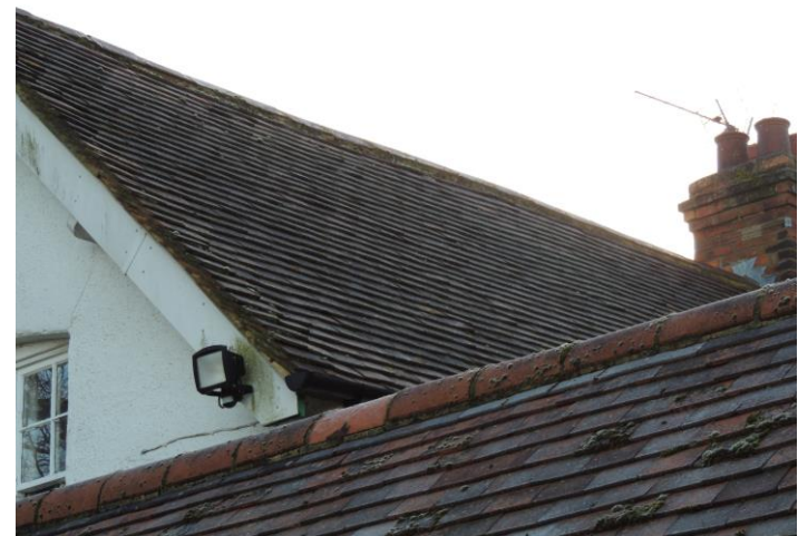
Photo 12: Note tight seal to roof tiles
