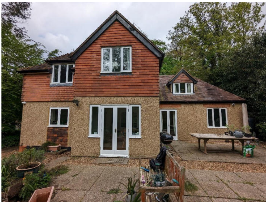
Fig. 3 – Photograph taken from the south east of the south east (rear) elevation of the dwelling
