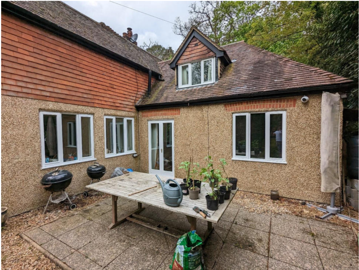
Fig. 4 – Photograph taken from the east showing the location of the proposed extension
