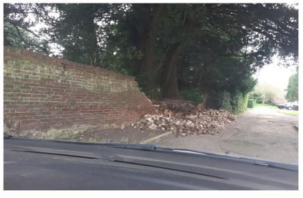
Following the collapse of a section of boundary walling which separates parkland at Barham Court from Woodlands Close Teston it has been established that the cause for the collapse was a horizontal thrust from an adjoining mature Holm Oak tree. The Holm Oak is considered to be in good condition and the tree is
