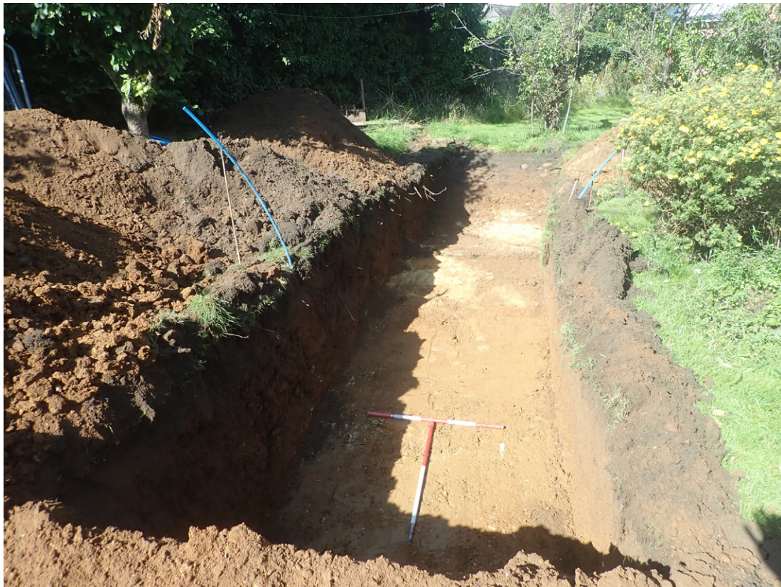
Fig. 3.2: Trench 2, facing north-west
