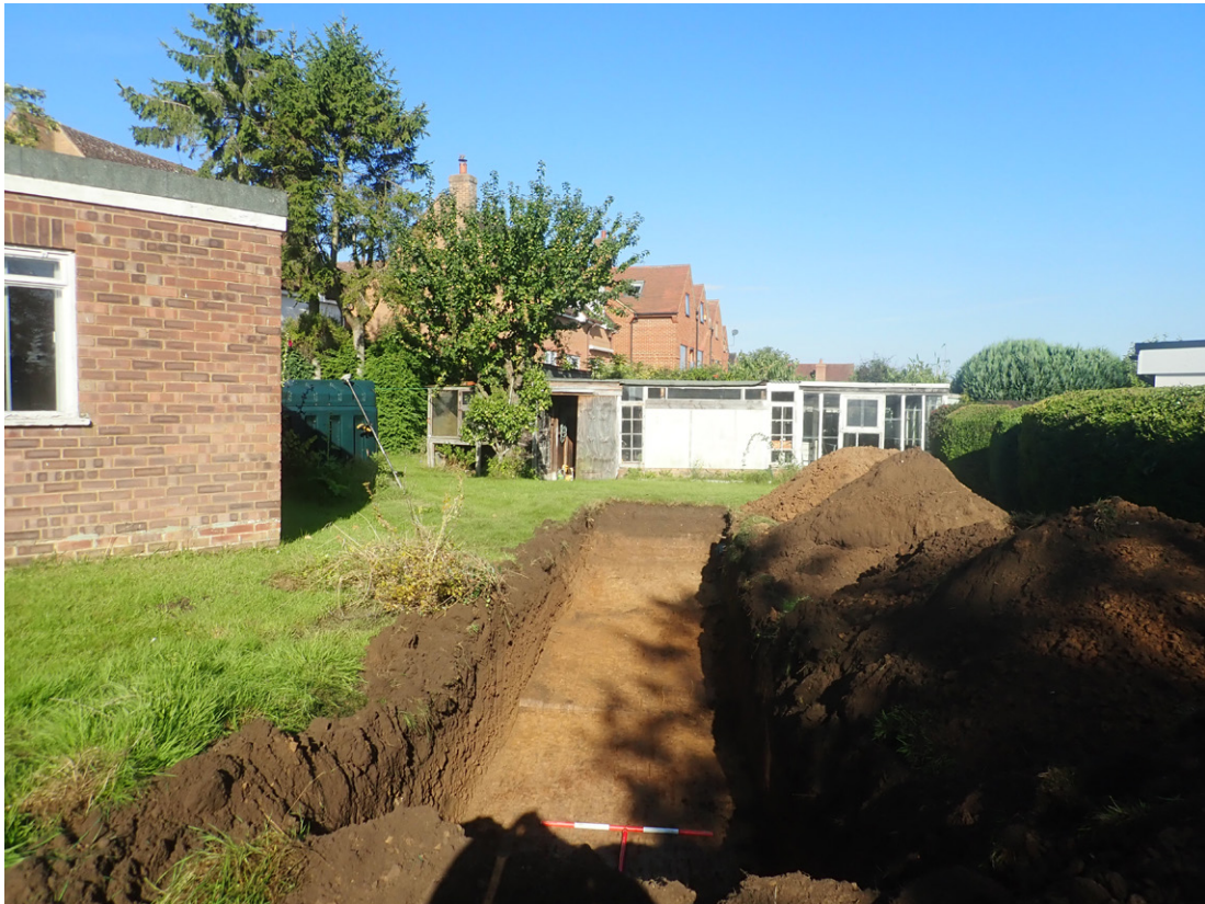
Fig. 3.1: Trench 1, facing north
