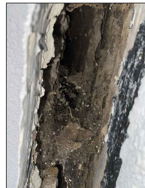
Exposed Timber Frame
