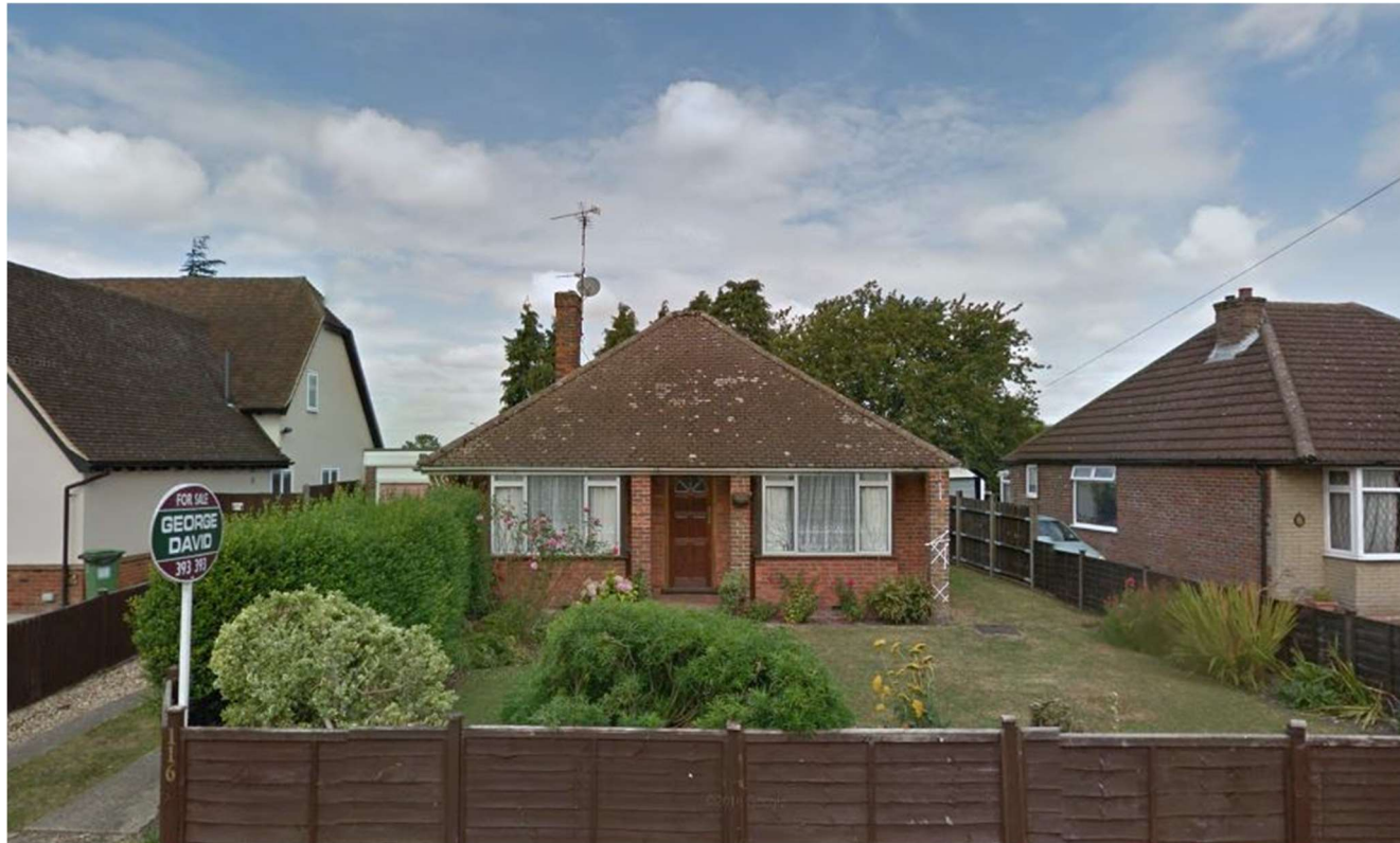
116 Weston Road, Aston Clinton, Aylesbury, HP22 5EP
