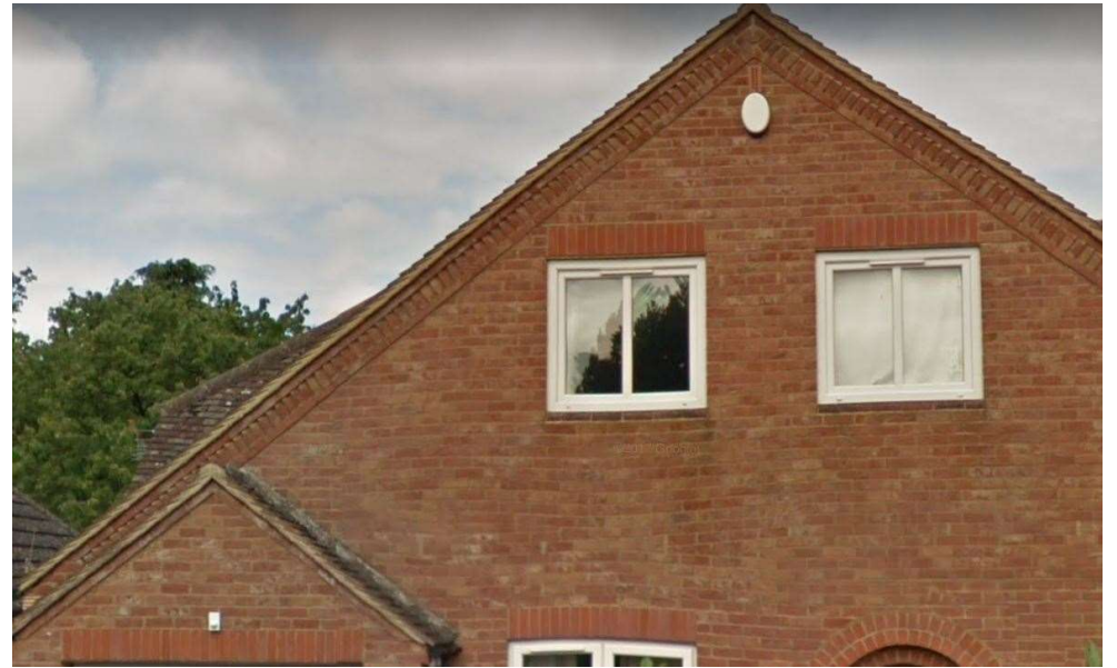
112 Weston Road – Decorative brick
