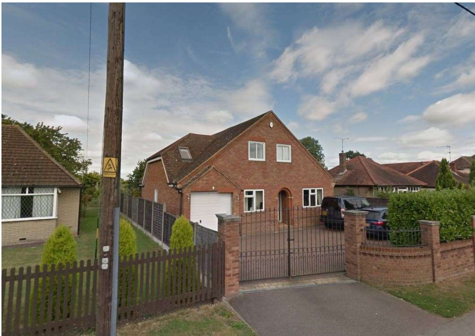
112 Weston Road – Brick detailing
