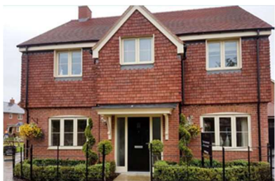
Precedent house taken from Aston Clinton design guide; our proposal shows the use of different materials and gable projection to break the elevation as in this example.
