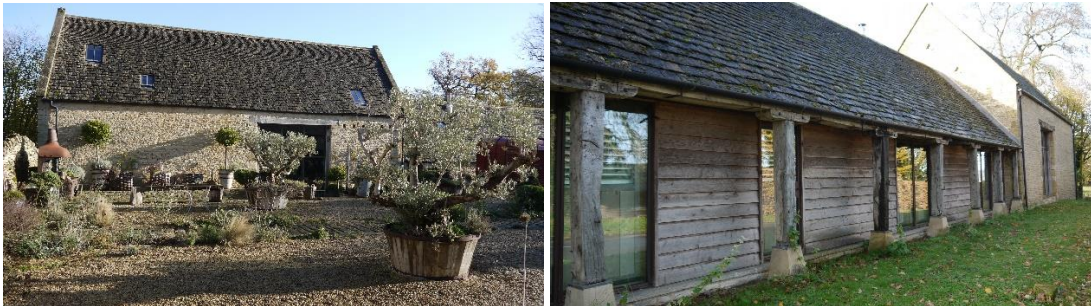
Plate 5 (left) Primary elevation of threshing barn, and Plate 6 (right) roadside elevation with new timber cladding and glazing.
