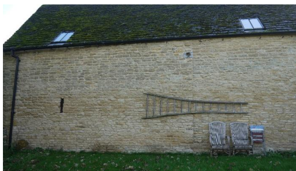
Plate 13 Rear façade and proposed area for new opening.
