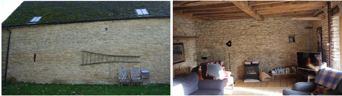
Plate 7 (left) Rear elevations of the former stables and vertical section showing two phases of construction and Plate 8 (right) internal image with exposed stone walls and timbers.
