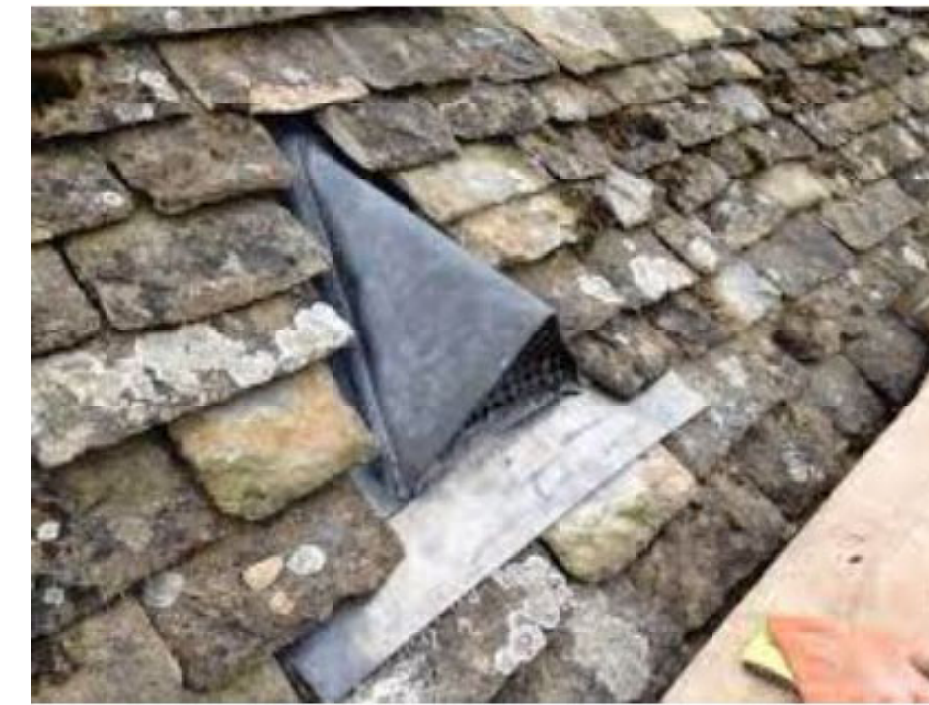
Lead vent to Cotswold stone roof for new bathroom extract
