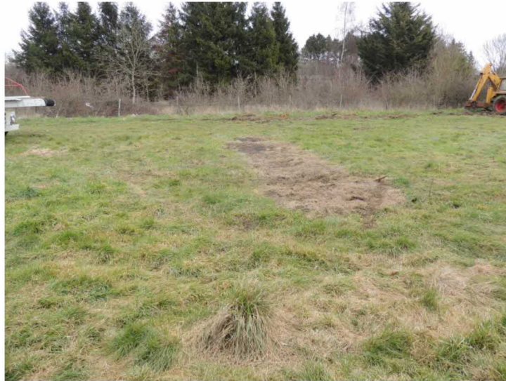
Photo 9: Looking SW-NE across the site
