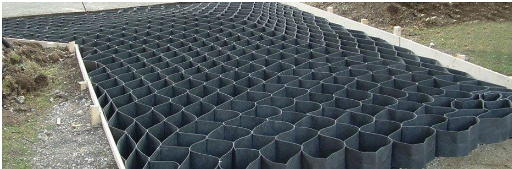
Figure 3 - Example 3-d cellular confinement system prior to installation of stone.
