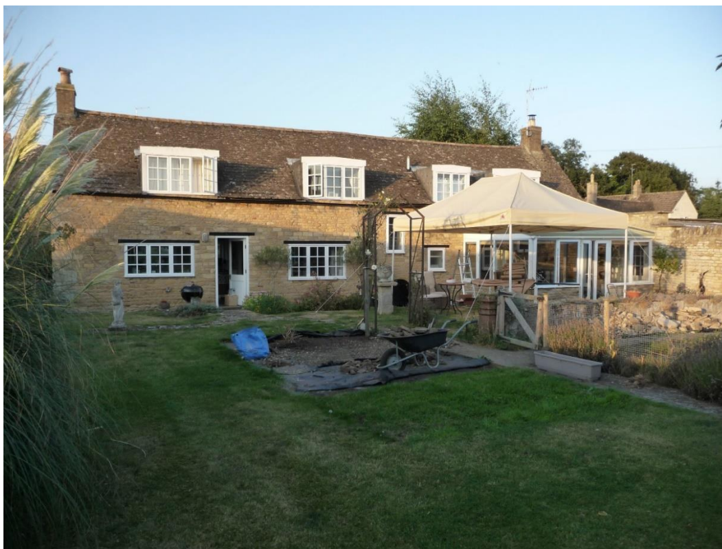
Figure 3. The rear of the house today. All the fenestration dates from the 1970s. The windows to either side of the door are very wide, and were probably extended.
