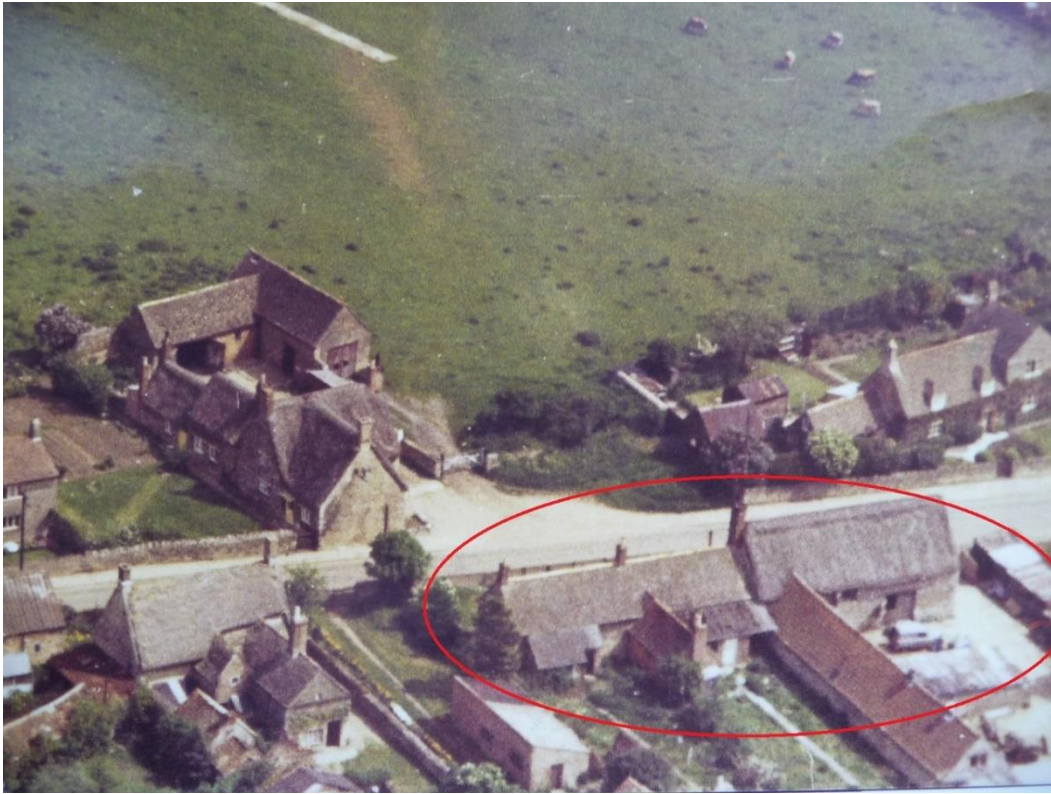
Figure 2. 1970s air photo showing the house (ringed, on the left) with no rear dormers.
