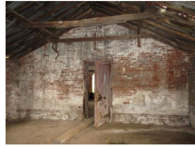
Interior of shed G: Left: looking E showing boarded up entrance with pedestrian door; Centre: looking W showing E former exterior wall of barn A with ventilation slits above inserted door; Right: N wall, raised in height with inserted window
