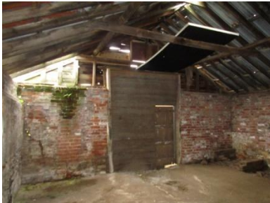
Interior of shed G: Left: looking E showing boarded up entrance with pedestrian door; Centre: looking W showing E former exterior wall of barn A with ventilation slits above inserted door; Right: N wall, raised in height with inserted window
