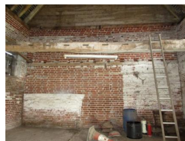
Left: NE corner of stable B, looking upwards showing binding beam and remains of ladder stair to loft on E wall beside loading hatch; Centre: Stable B looking S showing wall where doorway into proposed dining room; Right: N wall of stable showing lime washed area behind ladder where doorway is proposed in re-built 19th century brickwork
