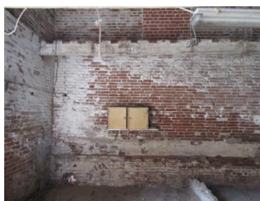
Left: NE corner of stable B, looking upwards showing binding beam and remains of ladder stair to loft on E wall beside loading hatch; Centre: Stable B looking S showing wall where doorway into proposed dining room; Right: N wall of stable showing lime washed area behind ladder where doorway is proposed in re-built 19th century brickwork
