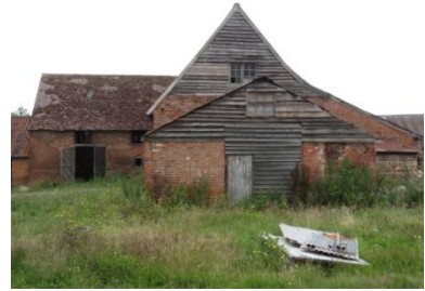
Left: E elevation of stable (B); Centre: E elevation mid-19th century shed (D) attached to stable; Right: E elevation of barn (A) showing boarded gable and attached early 19th century shed (G)
