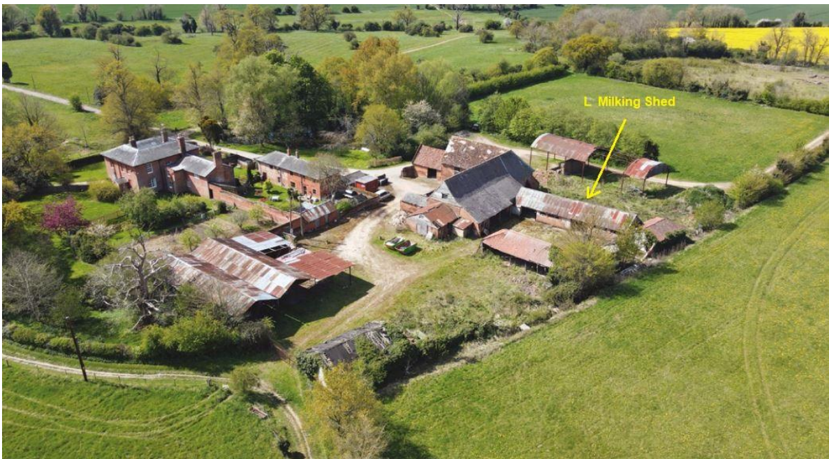
June 2008 Oblique aerial looking SW showing milking shed (proposed for partial removal) attached to N elevation of barn A
