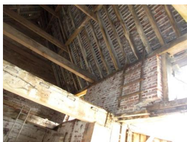
Left: NE corner of stable B, looking upwards showing binding beam and remains of ladder stair to loft on E wall beside loading hatch; Centre: Stable B looking S showing wall where doorway into proposed dining room; Right: N wall of stable showing lime washed area behind ladder where doorway is proposed in re-built 19th century brickwork
