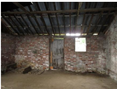
Left: interior of shed G looking S showing poor quality brickwork; Centre: looking S showing entrance to 20th century shed K attached to E wall of building J; Right: looking SW showing G, K and J attached to barn A
