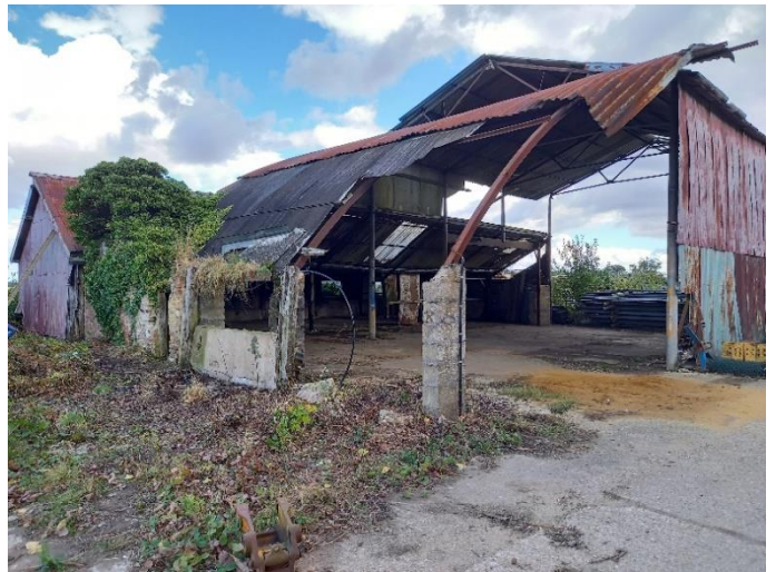
Photo 4 West end of B1 and south and west views of B3
