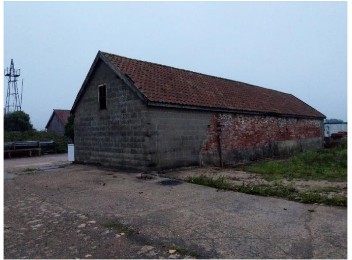
Photo 2 South and west elevations of barn B2
