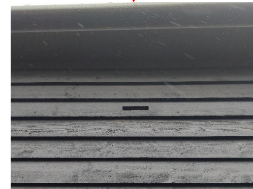
Access to the bat boxes cut into the weather boarding. The holes can be cut by scalloping the underside of the board where it covered the board below to reduce water ingress
