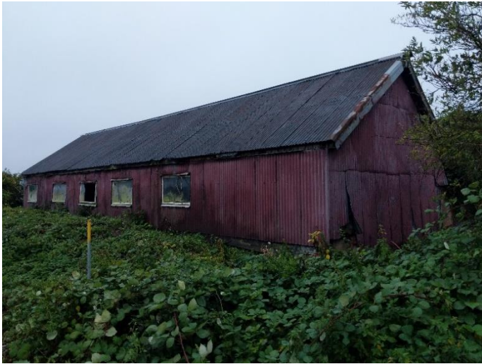
Photo 1 North and west elevation of single storey B1
