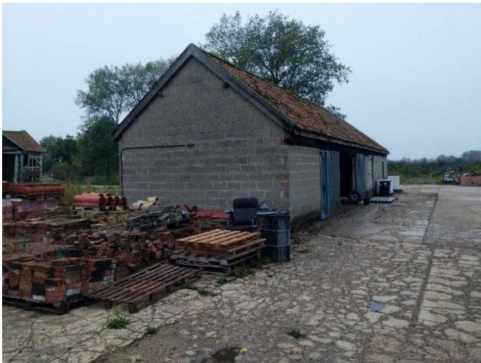
Photo 3 North and east elevations of barn B2
